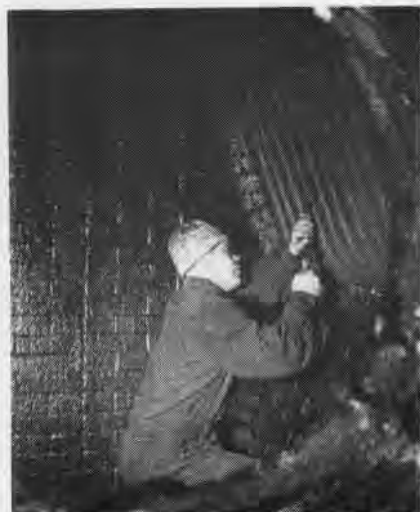
W. C. GILES CLEANS FIRESIDES OF A BOILER
