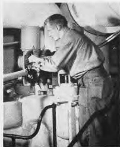
STEAM CONTROL VALVE ON ENGINE REPAIRED
