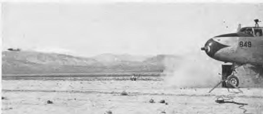
**Three cameras** on the ground and atop the plane fuselage record the flight of a 5" spin stabilized aircraft rocket as it leaves one of the twin launchers in the nose of this B-25 on the ground at NOTS Inyokern, Cal. Rate of fire is 300 a minute, with the fiery blast from the rockets being diverted by a tube downward out of the fuselage. Studies are also being made for shooting such rockets from rapid-fire installations in the plane wings.
