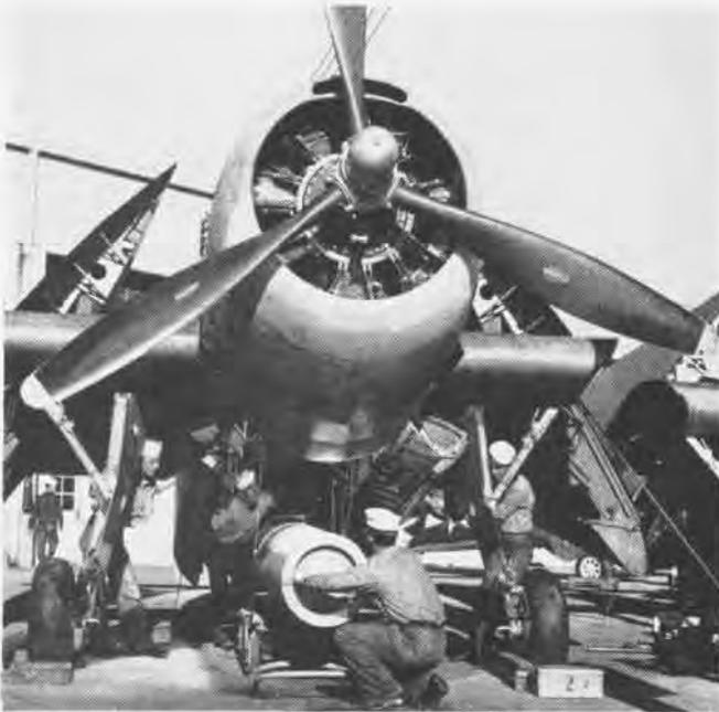
LEARN BY DOING—LOADING A TORPEDO INTO THE BOMB BAY OF A TBM
