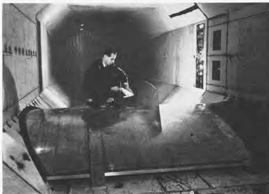
A method of obtaining controlled, measurable wind speeds in the transonic speed zone is claimed by Lockheed Aircraft Corporation. Through the use of this wind tunnel "bump" invented by John H.
