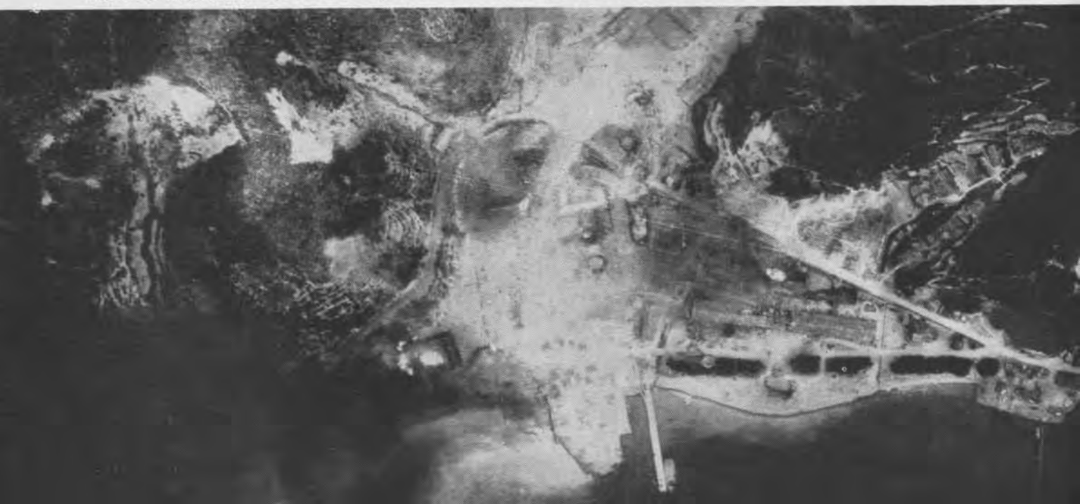
REVETTED AMMUNITION BUILDINGS (LEFT) BLAZE AFTER CARRIER PLANE ATTACK ON KONIYA SEAPLANE STATION AT AMAMI O SHIMA
