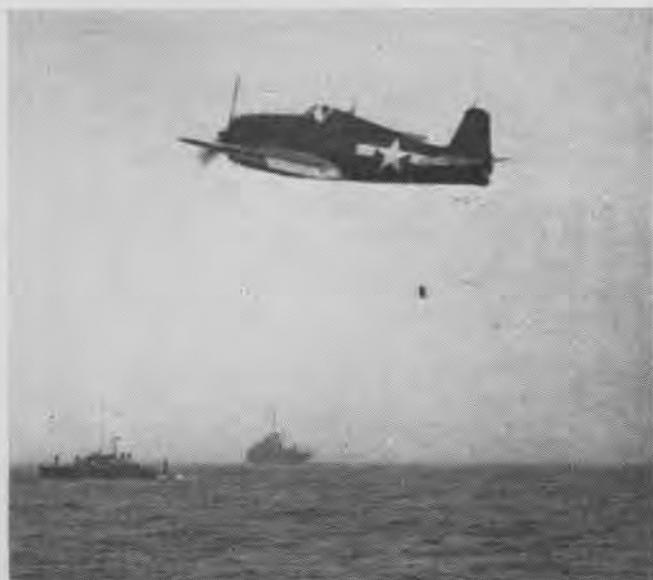
*Hellcat* rescue pilot releases first unit of original experimental AR-1 assembly from 50 to 100 ft. Assembly was stowed in cockpit
