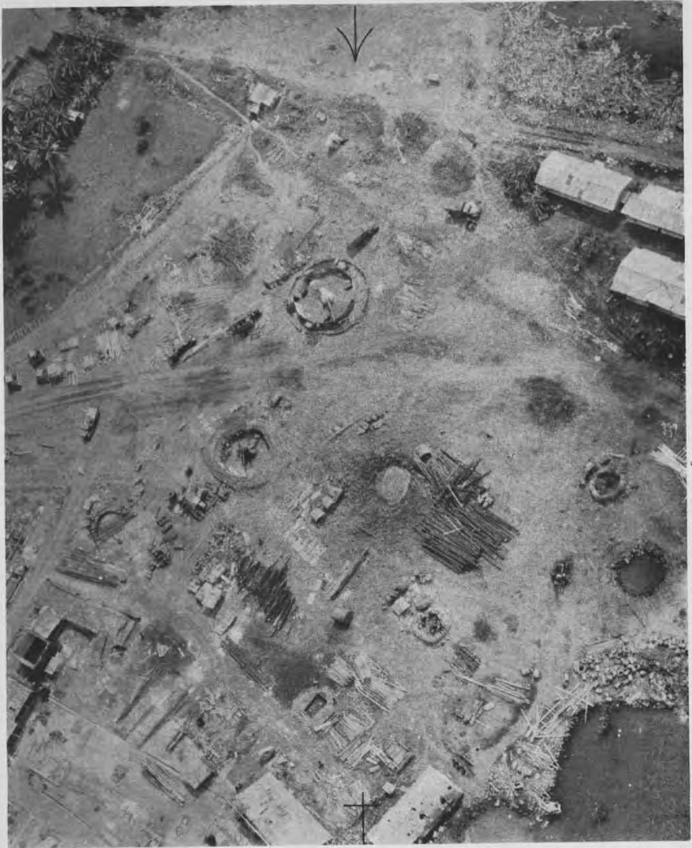
This low oblique taken by a Navy plane during an attack on Jap-held Truk presents varied information to the photo interpreter's analytical eye. Gun positions show typical construction with revetments. The scene is a center of construction activity with various building materials in piles. Stacks of prefabricated wooden trusses are to be used to roof various structures. Narrow gauge railways run into the
