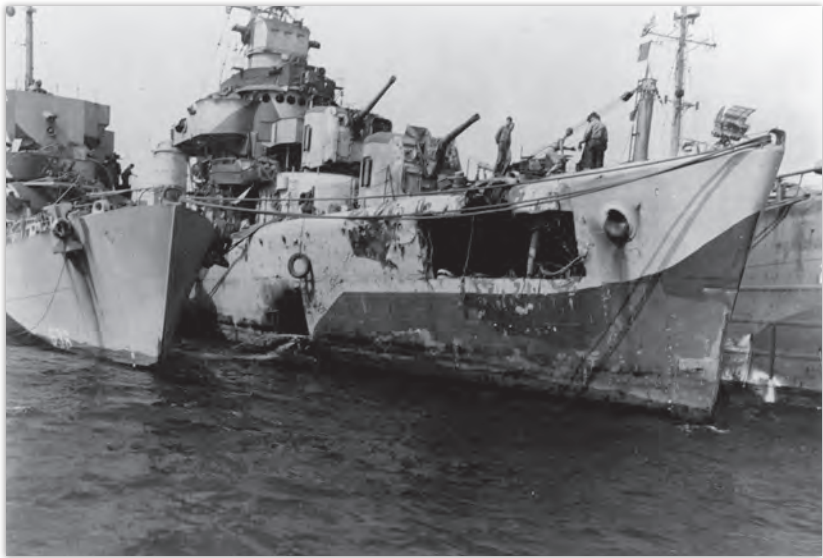
Destroyer minesweeper Rodman (DMS-21) and destroyer escort Witter (DE-636) undergo repairs at Kerama Retto on 9 April 1945. Both ships received heavy structural damage from kamikaze attacks on 6 April, off Okinawa. (NHHC, NH 69111)
