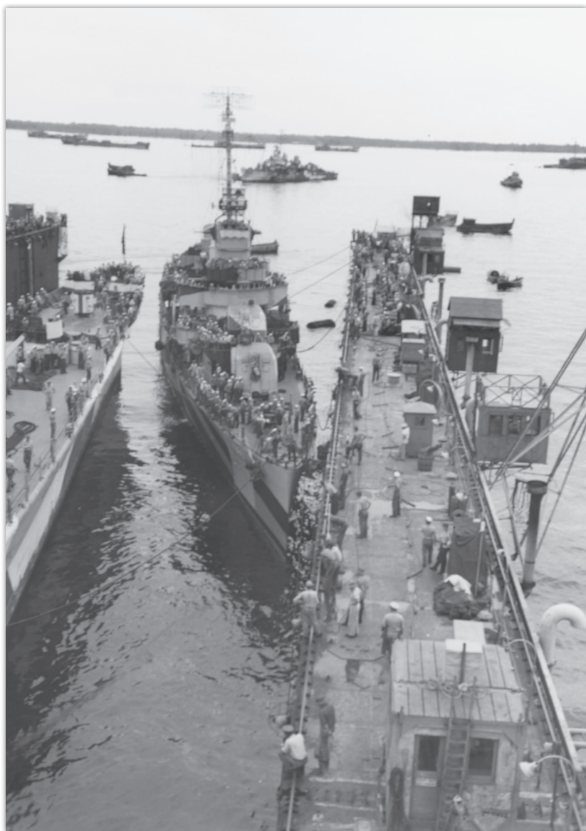
At Manus Island, Papua New Guinea, USS Claxton (DD-571) enters floating dry dock ABSD-2 in December 1944 for repairs. To Claxton's starboard is Canberra (CA-70). Kamikazes had damaged both ships. Killen (DD-593) appears in the center background, as well as a number of transports. By late 1944, the Navy's logistics apparatus had developed to provide mobile sustainment for naval forces, including the ability to complete repairs far forward, such as seen in this photograph. (NHHC, 80-G-359488)
