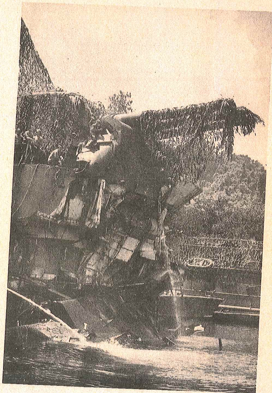
New Orleans at Tulagi after Battle of Tassafaronga. Bow is missing forward of Turret II
