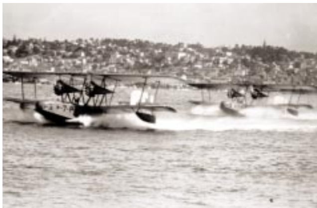
Two squadron PD-1s preparing to take off, note the Battle E on the nose of the second aircraft, 80-G-453499.
