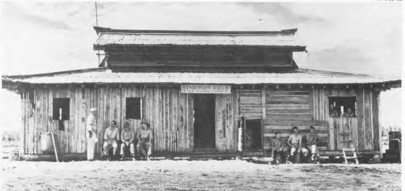
Marine and Navy air headquarters at Henderson Field. After surviving numerous Japanese bombings, this structure had to be torn down when a near miss rendered it useless.
