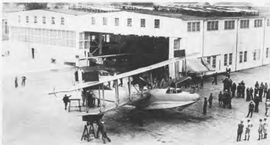
H-12 at an East Coast naval air station is readied for a flight prior to an antisubmarine sweep. The N-9 in the background was also used on occasion to patrol inshore waters.
