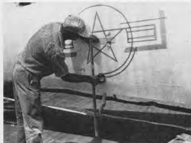
A MASK-TAPE dispenser applicator is a novel device designed by an employee at Naval Air Facility, Litchfield Park, Arizona. Mr. Nicholas L. Mandigo (Painter, Finish and Insignia), Maintenance and Preservation Department, entered the idea via the Navy Incentive
