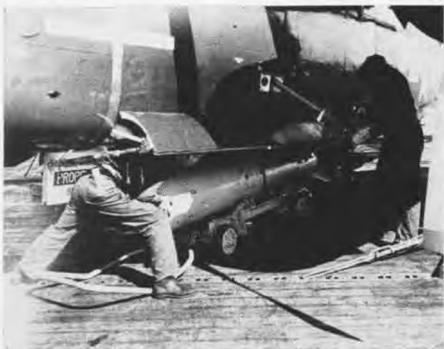
ORDNANCEMEN load homing torpedo. Fitted with dummy warhead for exercises, but no explosive charge, torpedo can seek out, strike sub.
