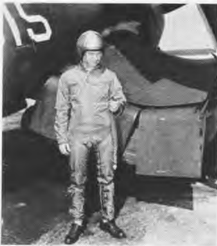
Deflated standard anti-G suit replaces the flight suit; pilot holds oral blowup plug.
