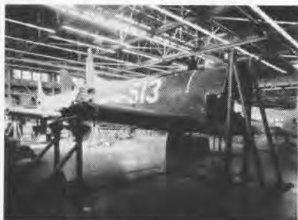
JIG SUPPORTS AD AIRCRAFT BEING REPAIRED
