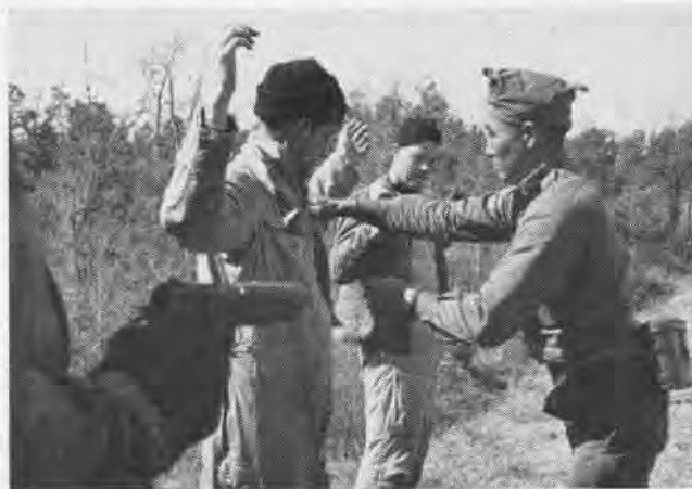
GUARD'S COCKED HAMMER INDICATED SERIOUSNESS OF CAPTURE
