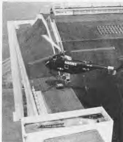
THE GEAR WAS DELIVERED IN FIVE TRIPS
