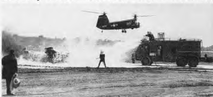
NEW EGGBEATER PRINCIPLE, SPECIAL PUMPS PRODUCE SNOWSTORM OF FIRE-KILLING FOAM
