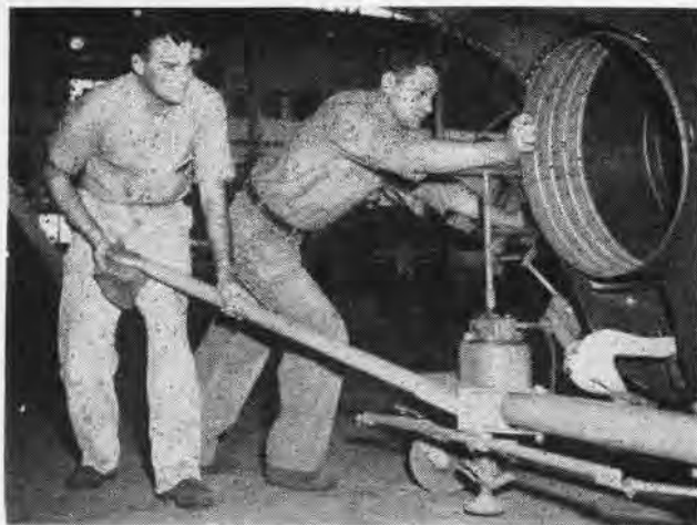
PLACING tail section on a tail-jack, V. C. Carnazza and A. J. Ferranti, AD1's, prepare to make acceptance check on Cougar.
