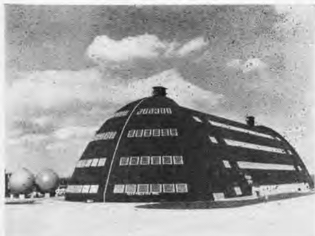
FORMER BLIMP hangar now houses former NAS Squantum reserve squadrons and dwarfs cars parked on hangar's ramp near door.
