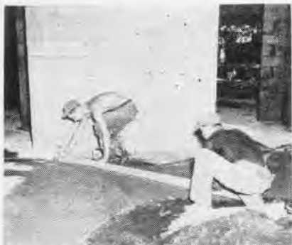
CONSTRUCTIONMEN level the concrete floor of Sangley's dependent housing unit.
