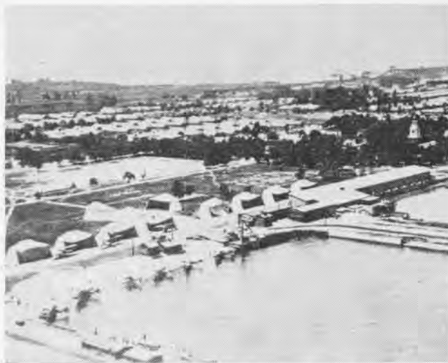
THIS IS the site of the original O&R. Land in the background, mostly marsh, has been filled in and is the location of the present runways.
