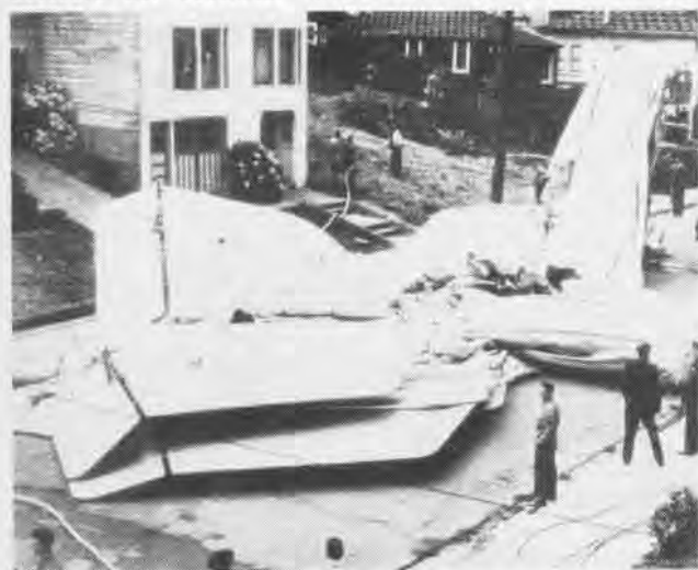
ENVELOPE LIES COLLAPSED AFTER BEING RUPTURED BY FIREMEN
