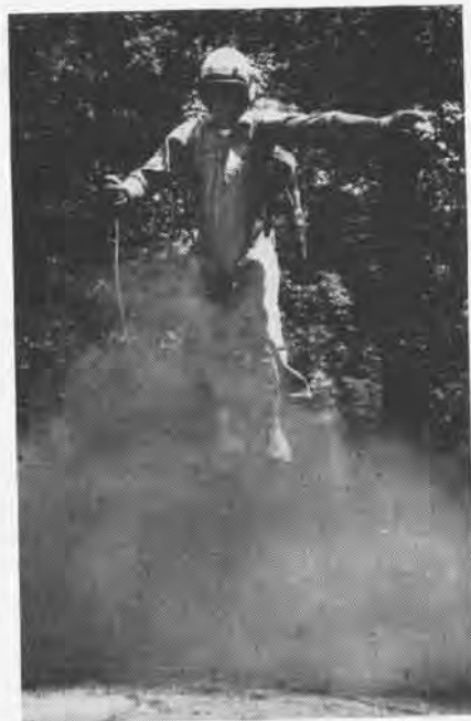
ROCKET-POWERED jump belt worn by soldier at left, developed by Reaction Motors Division of Thiokol Chemical Corporation, might enable troops to achieve an element of mobility they have never enjoyed. Ed Kurczewski, Test Stand Assistant for Reaction Motors, demonstrates a power-assist leap at right, using an early version of the jump belt. He carried equipment weighing approximately 30 per cent of his own weight, yet vaulted to distance of 20 feet.
