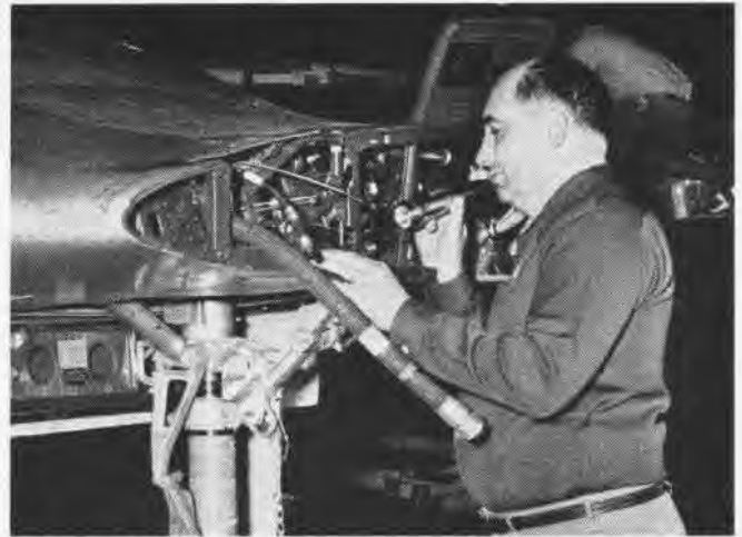
Inspector Andrew Jenkins is inspecting a center wing panel assembly of an aircraft at the end of the center section assembly line
