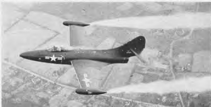
PANTHER JETTISONS GASOLINE FROM ITS NON-DROPPABLE WING TANKS, LEAVING VAPOR TRAIL
