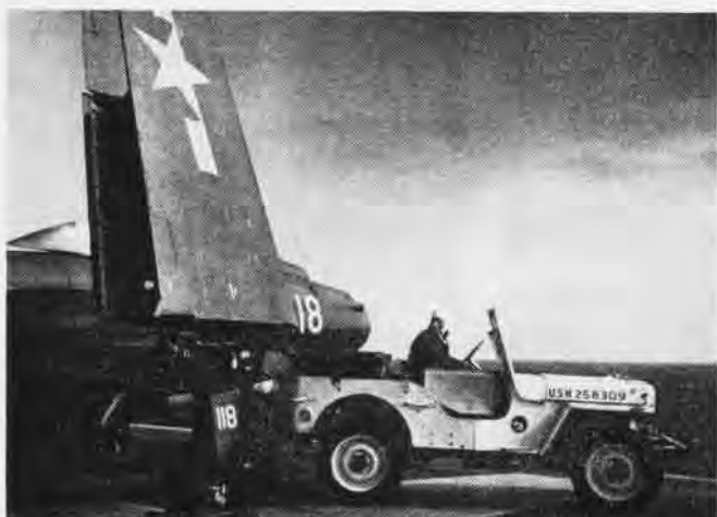
Eight batteries in jeep provide starting power for Phantoms which require external energy to start their 19XB engines
