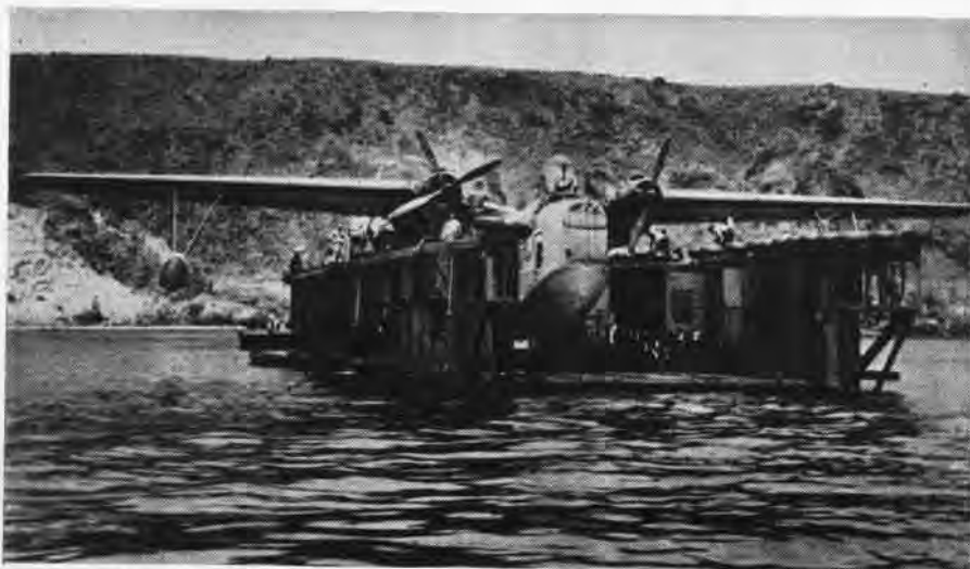
DRYDOCK RAISED TO FULL HEIGHT PROVIDES FACILITIES FOR MAINTENANCE WORK ON SEAPLANE
