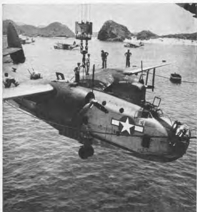
Kerama Retto in Ryukyus forms background for this view at a seaplane base. Aboard a barge, PBM will get routine repairs
