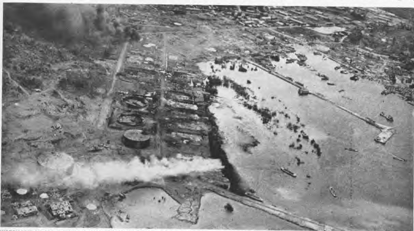
WRECKAGE OF JAP OIL TANKS AND DUBLON TOWN IN TRUK ATOLL SHOWS HEAVY DAMAGE DONE BY RAIDING PLANES FROM CARRIERS
