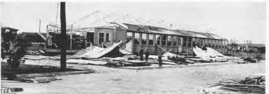
TWO BUILDINGS WERE RIPPED APART BY THE WIND. MANY OTHERS WERE BADLY DAMAGED
