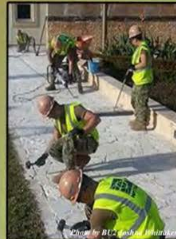
Photo by BU2 Joshua Whitaker SOUDA BAY, Greece - Crew members from Public Works Department Souda Bay, Greece builder shop prepare concrete surface at Building One for the placement of tile.
