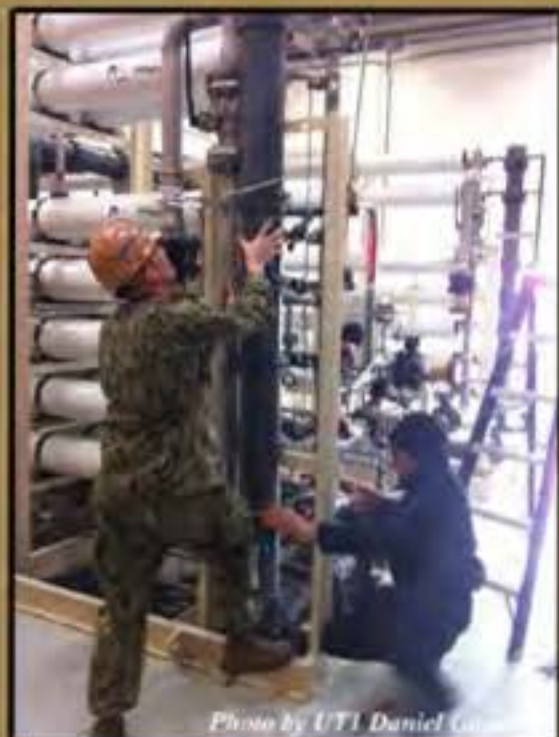
Photo by UTI Daniel Guzman SIGONELLA, Sicily - Utilitiesman Constructionman Apprentice Ryan Brooks and Fabio Calabrese of the Public Works Department Sigonella, Sicily plumbing shop begin the replacement of a ruptured six-inch PVC pipe at Naval Air Station Sigonella water treatment plant's permeate line.
