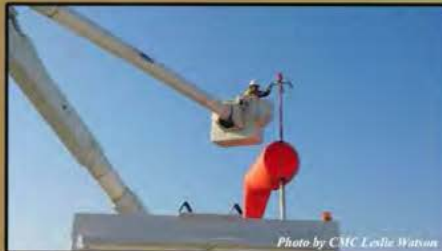
Photo by CMC Leslie Watson ROTA, Spain - Construction Electrician 3rd Class Daniella Acevedo of Public Works Department Rota, Spain inspects runway approach lighting on board Naval Station Rota in order to ensure continued flight operations.
