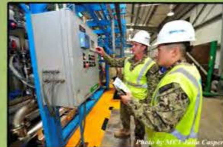
Photo by MC1 Julia Casper CAMP LEMONNIER, Djibouti - Lt. Nathan Chenarak (right) and Utilitiesman 1st Class Waverly Holland (left) spot check flow and pressure readings on the Reverse Osmosis Water Purification Unit (ROWPU) plant at Camp Lemonnier, Djibouti, Africa. The ROWPU produces 250,000 gallons of fresh drinking water per day for the residents of Camp Lemonnier.
