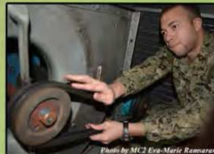
Photo by MC2 Eva-Marie Ramsaran NAPLES, Italy - Machinist's Mate 1st Class Gregory Rochester of Public Works Department Naples, Italy replaces an air supply pump motor belt for the air handler units at Naval Support Activity Naples Feb. 4, 2015.
