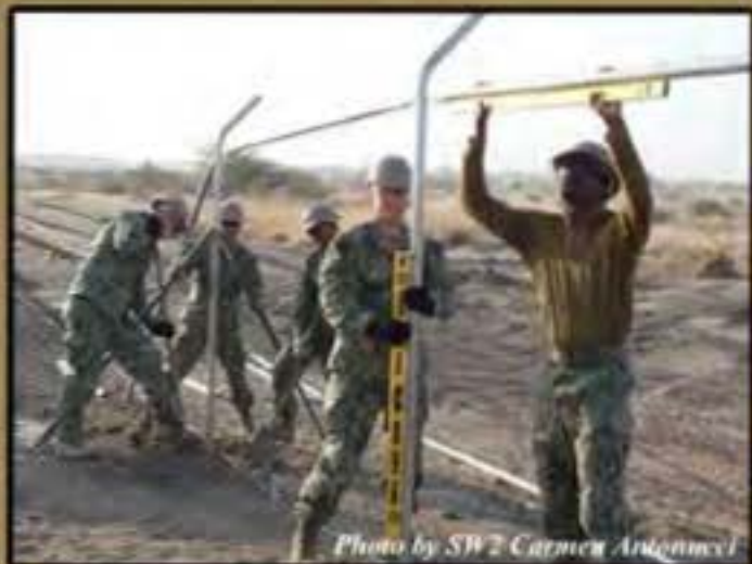
Photo by SW2 Carmen Antonucci N'DJAMENA, Chad - Naval Mobile Construction Battalion 14 Seabees place and level a security fence, Jan. 25, 2015, in support of Exercise Flintlock 2015.
