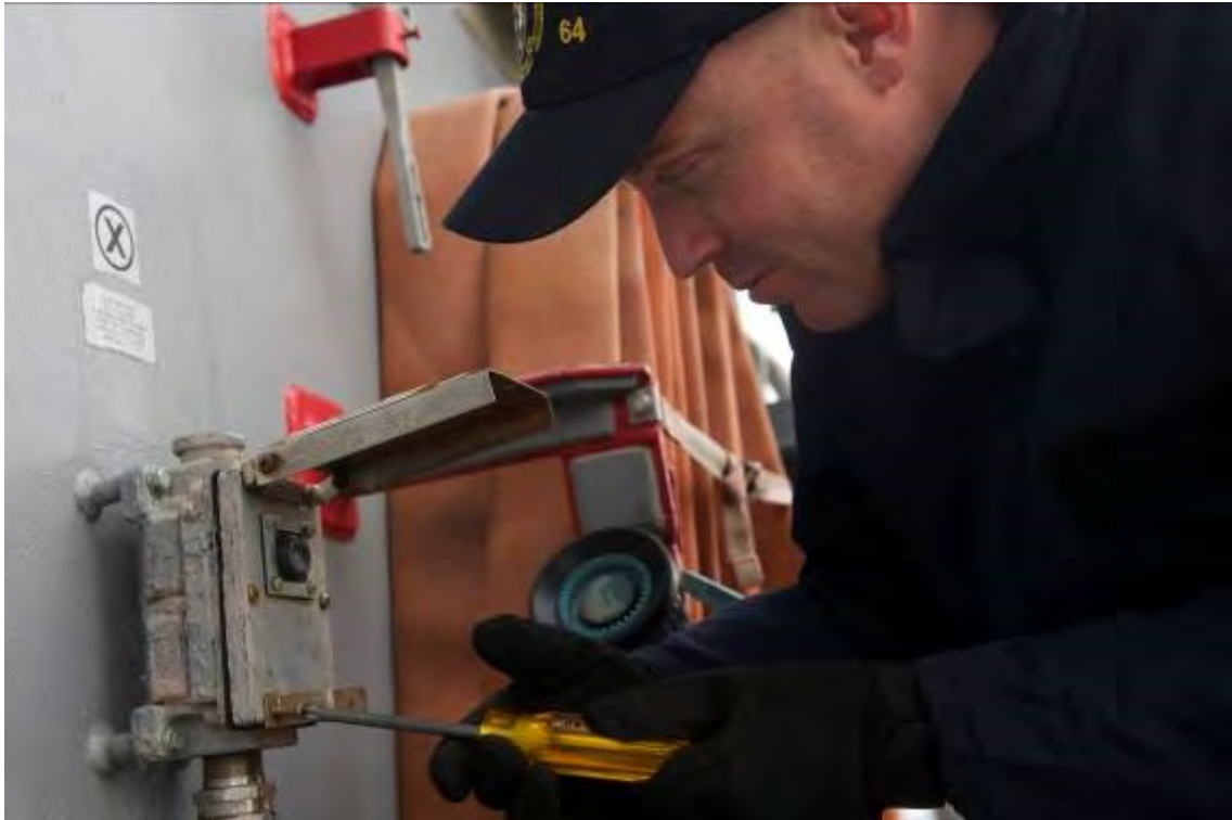
SOUDA BAY, GREECE (Jan. 18, 2016) Electricians Mate 2 nd Class Tuart Compton from San Diego, replaces an Aqueous Film Forming Foam (AFFF) emergency switch aboard USS Carney (DDG 64) Jan. 18, 2016. Carney, an Arleigh Burke-class guided-missile destroyer, forward deployed to Rota, Spain, is conducting a routine patrol in the U. S. 6 th Fleet area of operations in support of U.S. national security interests in Europe. (U.S. Navy photo by Mass Communication Specialist 1st Class Theron J. Godbold/Released)
