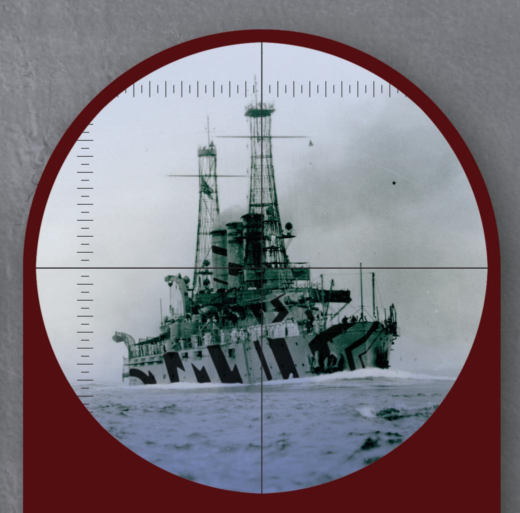
Razzle Dazzle camouflage made it difficult to determine which side of the ship the observer was seeing by distorting the apparent position of distinct parts of the ship. Until the ship came near enough for the observer to see through the camouflage, it was almost impossible to accurately judge the target's heading.
