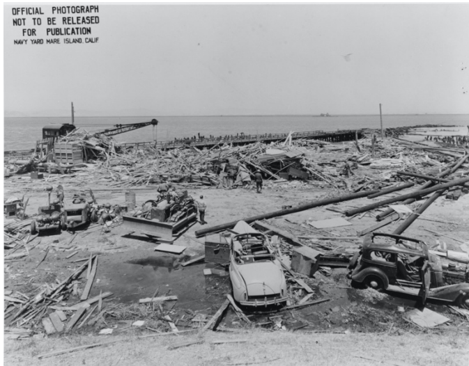
Naval Magazine, Port Chicago, California: Damage resulting from the 17 July 1944 ammunition explosion. This view looks north, showing the wreckage of Building A-7 (Joiner Shop) in the center and the destroyed ship pier beyond. Note bulldozer and damaged automobiles in the foreground, railway crane at left, and scattered pilings (NH 96823).
