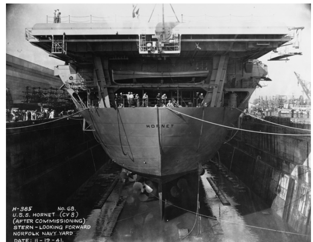
USS Hornet (CV-8): View taken after commissioning at Norfolk Navy Yard, Portsmouth, Virginia, 19 November, 1941, from directly astern while in drydock. Note details of after end of flight deck, ship's name across stern, and ship's boat stowage beneath flight deck (19-N-26400).
