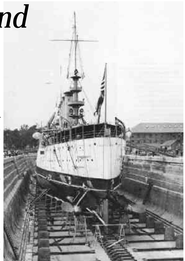
USS Maryland (ACR-8) is shown here breaking in the Navy’s newest drydock at the Charlestown Navy Yard in Boston, 1909. Built by Newport News Shipbuilding, she was one of the “Big Ten” series of fast armored cruisers constructed for the Navy shortly after the Spanish-American War. (U.S. Naval Institute photo)
