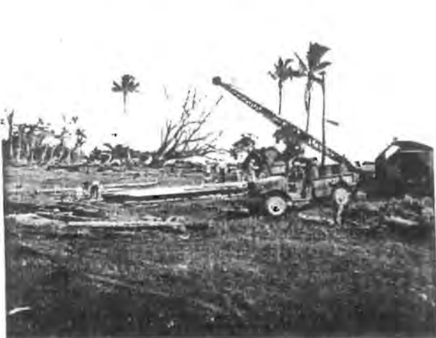
Laying the Foundation for a New Mess Hall
