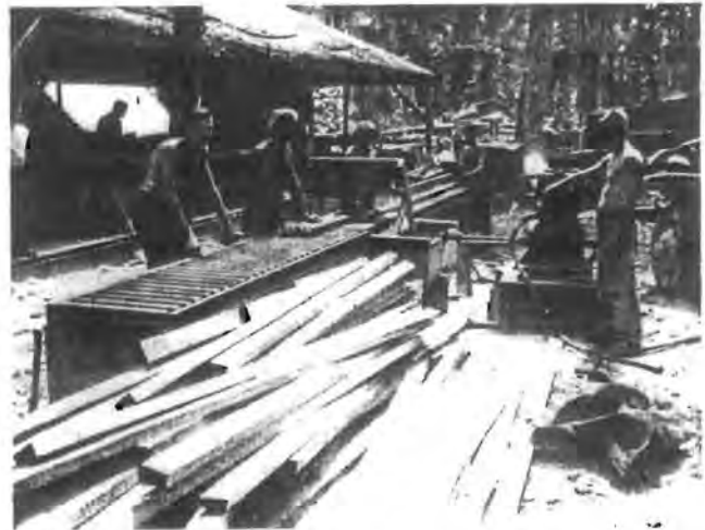
Jap Motor Powering a Home-made Saw
