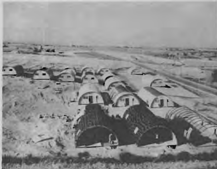
Hospital Unit, Mostaganem
