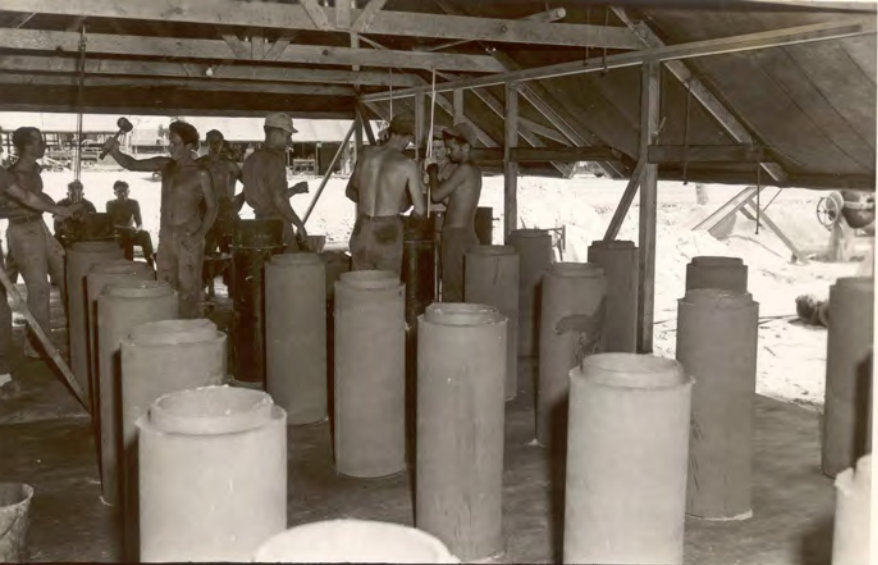
CONCRETE PIPE PLANT 25 TH N.C.B. SHOP AREA
