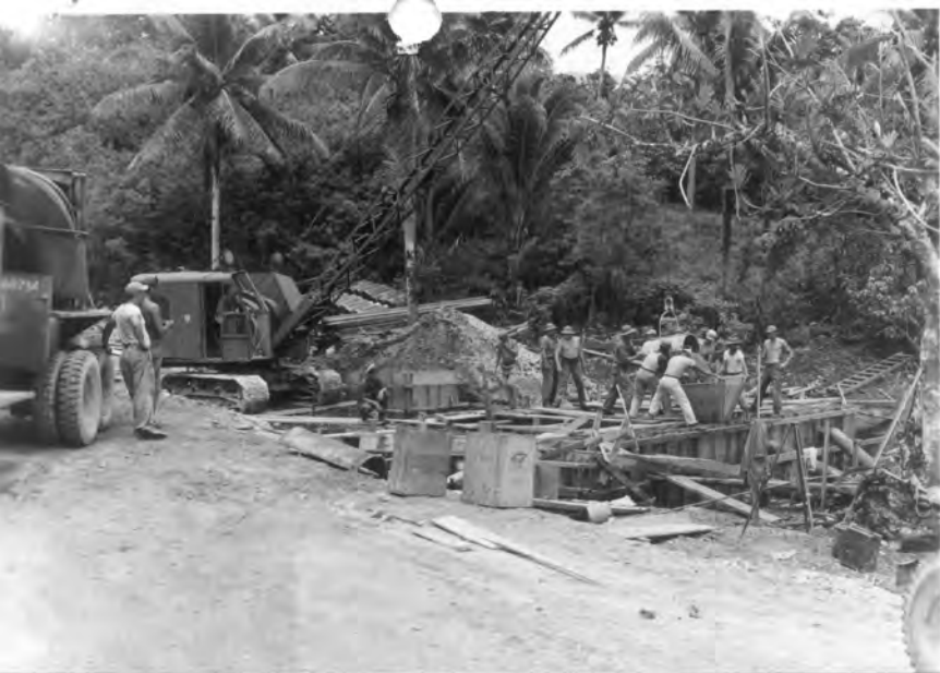
ADCOMPHIBSPAC CAMP AREA SEPTIC TANK
