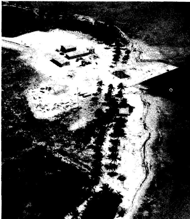
Typical outlying site. Eight of these sites are under construction, ranging from 20 to 150 miles from the Main Base. They are accessible only by aircraft or boat.
