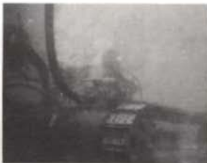
Divers used hand-held and tracked crawler pneumatic drills to drill dynamite holes for blasting out obstacles and leveling steep slopes along cable path. They also drilled holes in the rocky floor for placing U-bolt anchors to prevent cable motion and possible fatigue failure.
