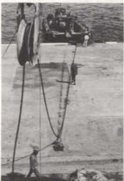
Tug assisted in-haul of cables from the cable tanks in the ships to the beach. Crawler tractors atop cliff on shore pulled cable to antenna sites.
