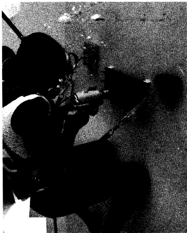
Magnets and tethering vest hold diver in place while hole is drilled.
