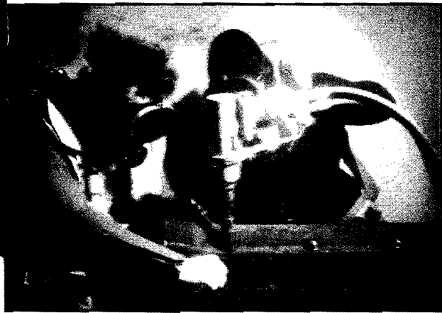
Two Seabees assemble split pipe with a hydraulically powered impact wrench.
