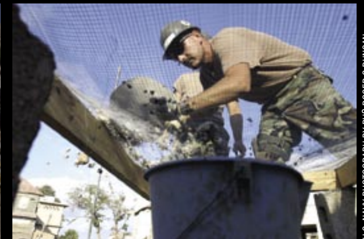
LEFT Seabees pour the foundation for a three-room school house at La Nativite School. RIGHT Navy Builder 2nd Class (SCW) Steve Byers, from Paintsville, Ky., sifts sand through a screen at a construction site in Gonaives, Haiti. The sand was used to make mortar that Byers and fellow Seabees used to build one of eight schools. The Seabees are assigned to NMCB 1 based out of Gulfport, Miss.
