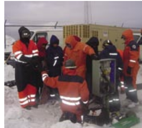
New installation is prepared
