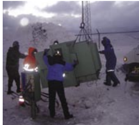
Broken transformer is removed
