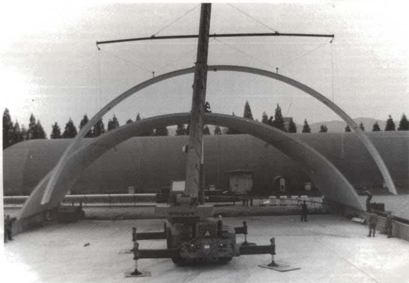
Members of NMCB 4's Detail For Training Korea use a crane to place a building section at a Super K-span project in Kwang-Ju, Korea. (Official Navy Photograph)
