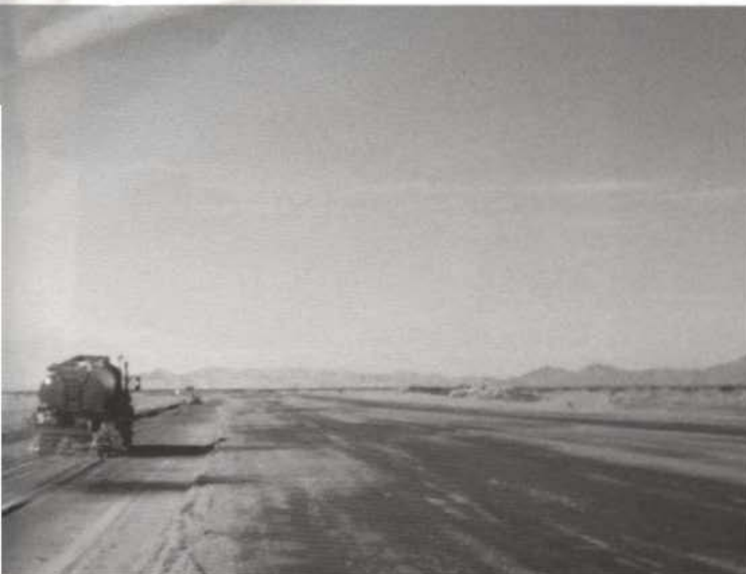
LEFT: A water truck plies the stretch of runway near the completion of the Aux II runway project, a joint refurbishing effort by Navy Seabees and Marines. BELOW LEFT: Tons of dirt were moved during the project. BELOW RIGHT: AC-130 glides towards the Aux II runway for an initial landing.
