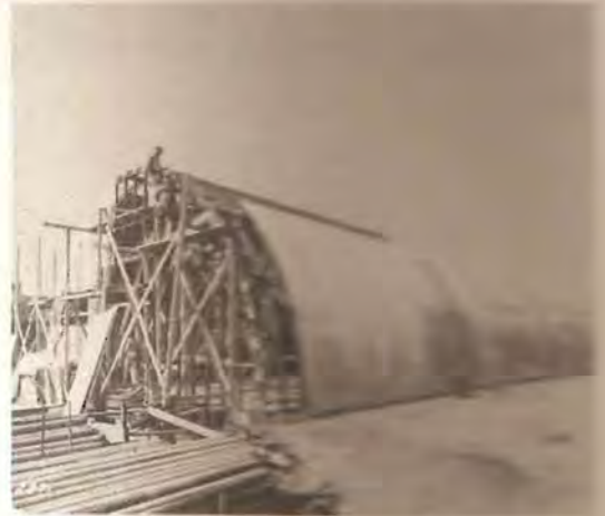
APPLY ROOFING SHEETS
