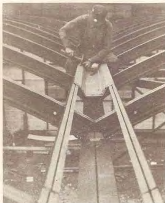
INSTALLING GUTTER
