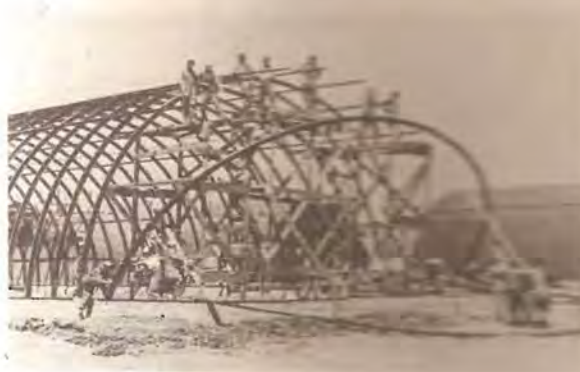
ERECT LAST RIB
