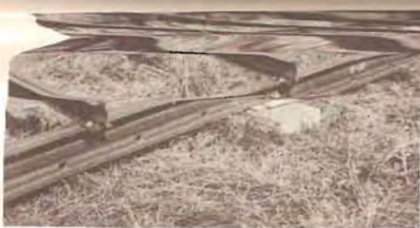
Floor joist assembly
