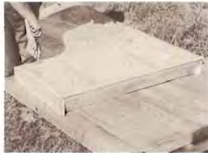
Place sash and attach hinges
