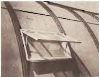
Nail the jamb clips into the ribs
