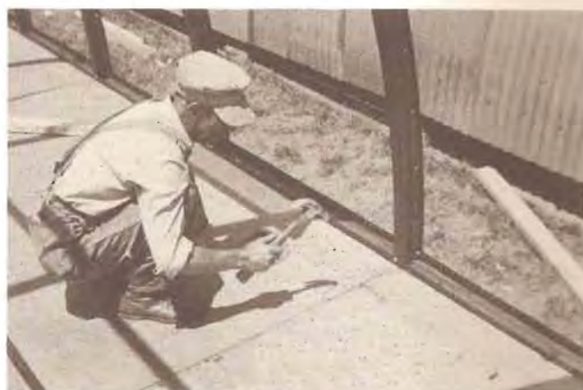
Nail panels in place
