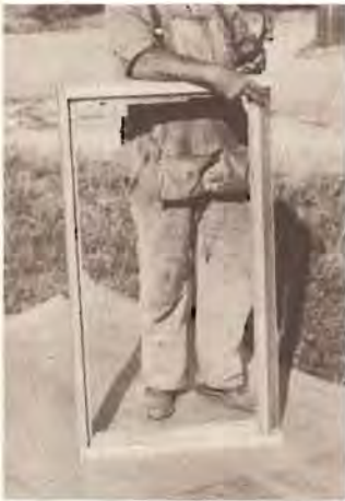
Assemble the knock down window frames
