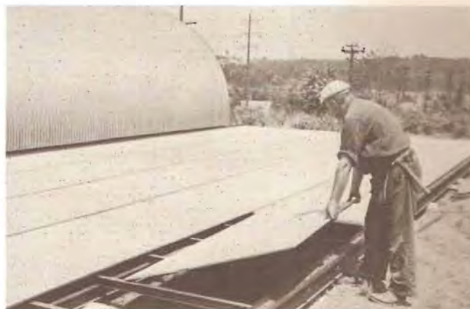
Lay-out plywood panels
