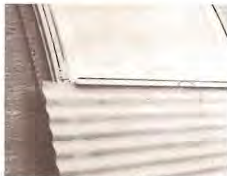
Drive one nail in valley of first corrugation
