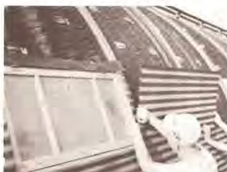
Between sheet and window place corrugated asphalt
