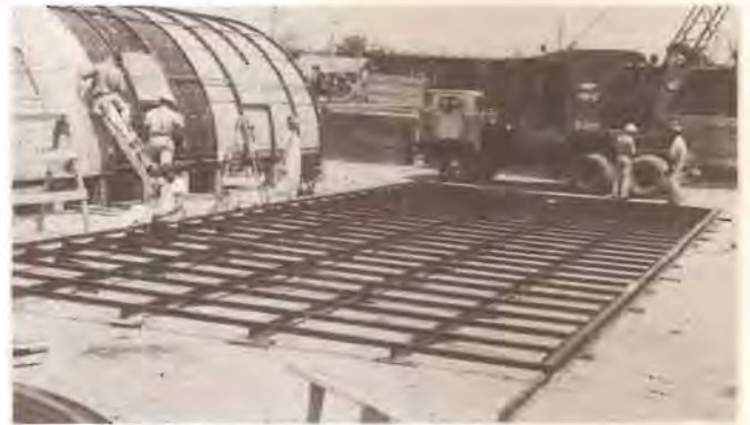
Complete joist assembly
