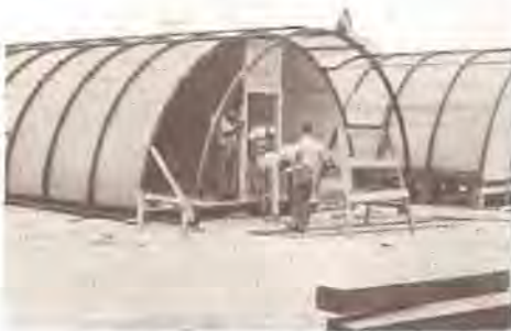
Place door frame in position
