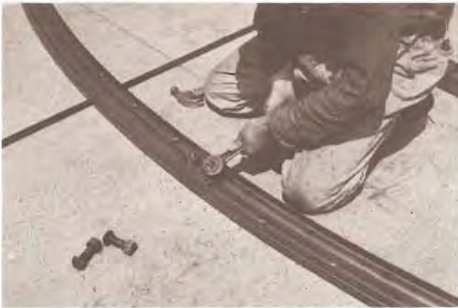
The half ribs are joined with the splice plate
