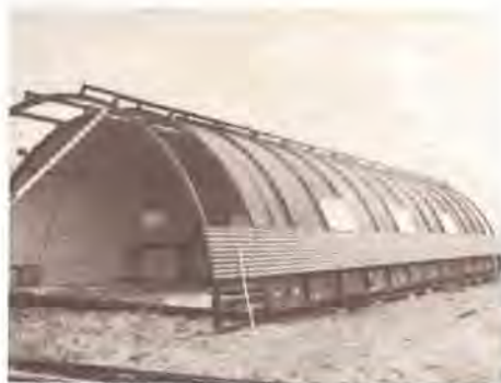
Start with row under window sill
