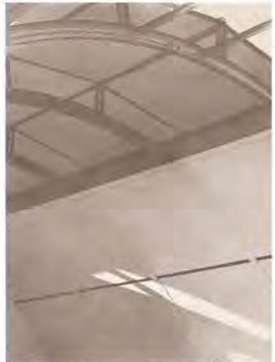
Nail "B" sheets to trimmers
