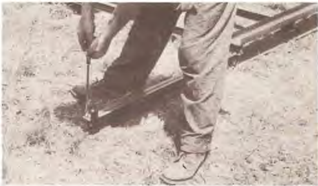
Screw rib shoe to sill
