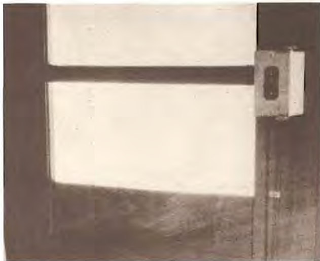
Fasten box to door jamb
