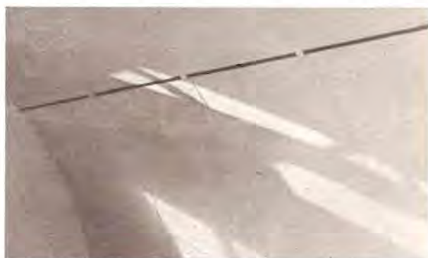
Metal splines between horizontal joints
