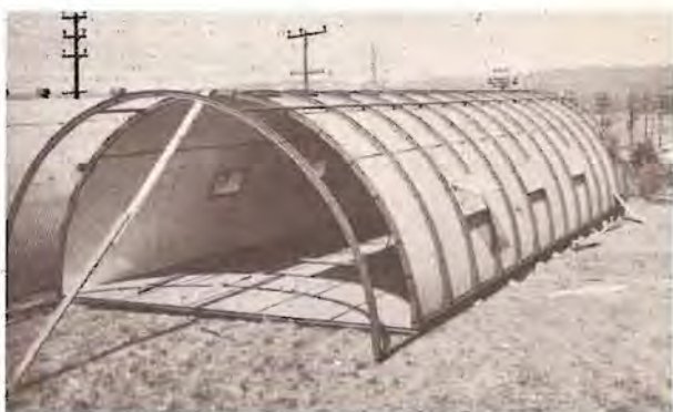
Inside covering installed
