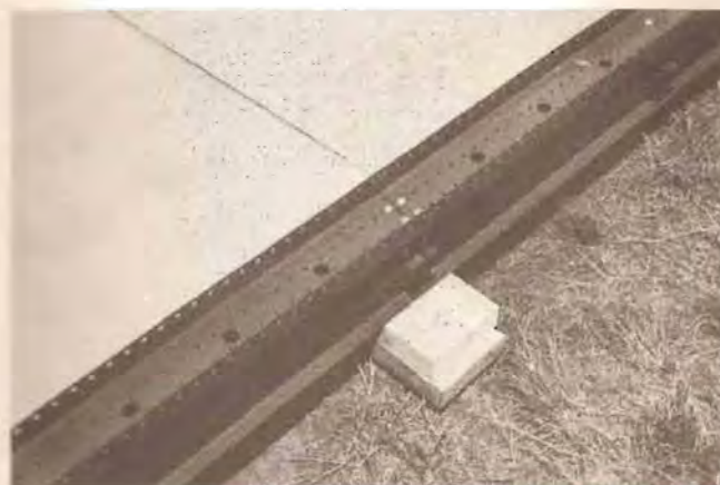
Panels butt over joist
