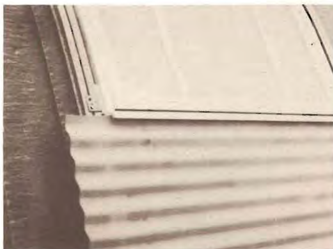
Fit insulation around windows
