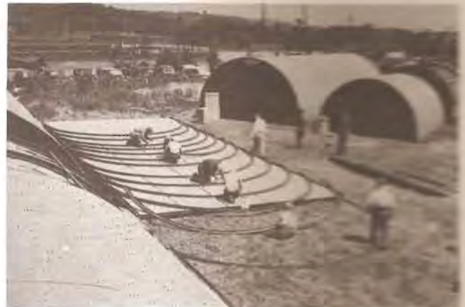
Assemble all the ribs on the floor
