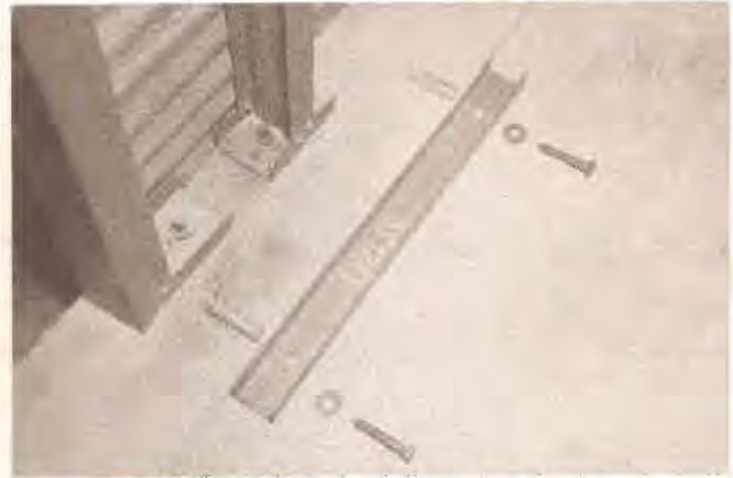
DOOR JAMB AND GUIDE CHANNEL
