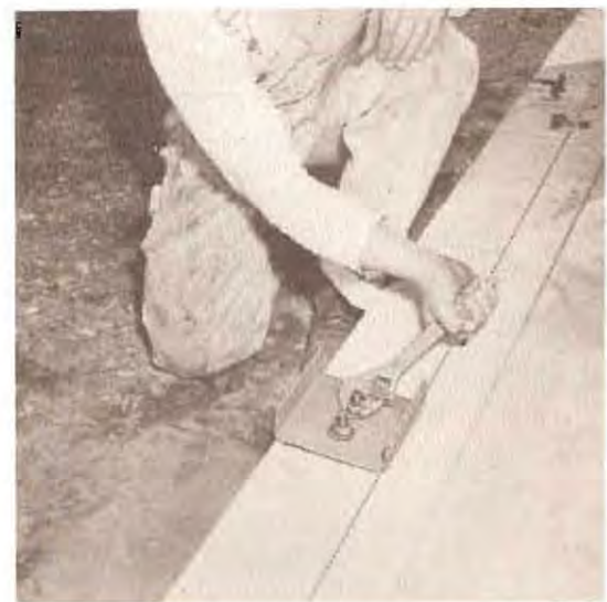
BOTTOM CHANNELS BOLTED DOWN
