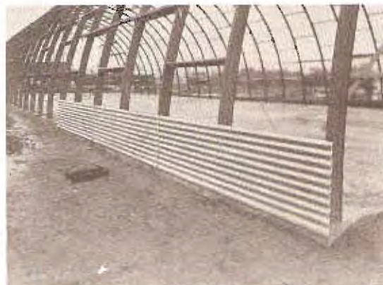
FIRST ROW OF SHEETS ON SIDE WALL
