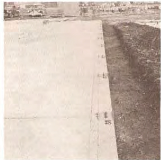
BOTTOM CHANNELS PLACED OVER ANCHOR BOLTS
