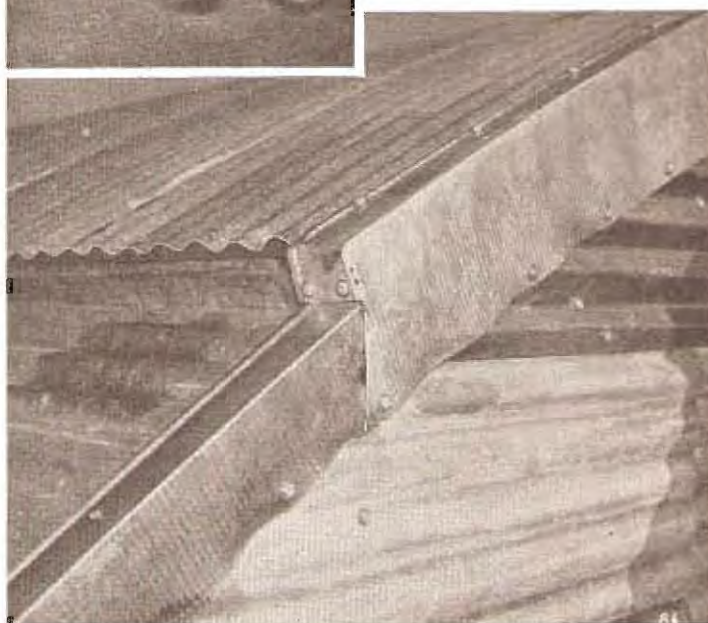
FLASHING DETAIL AT BULKHEAD
