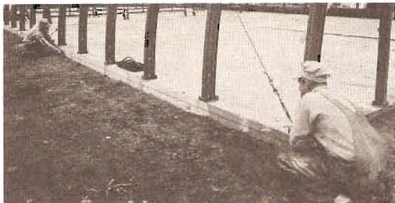
MARKING GUIDE LINE ON FOUNDATION FOR APPLYING SHEETS
