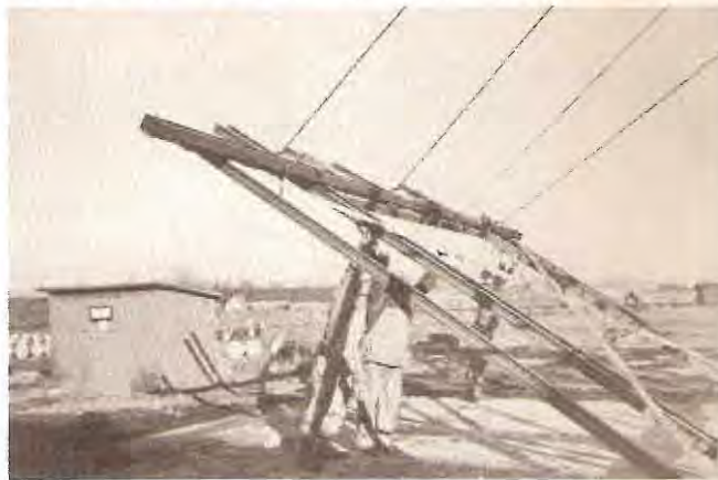
BULKHEAD FRAME HOISTED INTO POSITION
