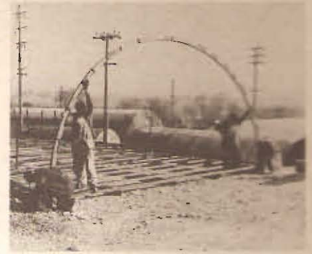
ERECT END RIB
