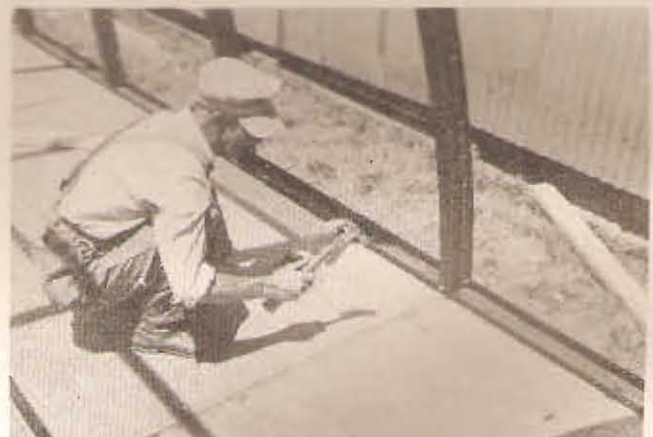
NAIL PANELS IN PLACE
