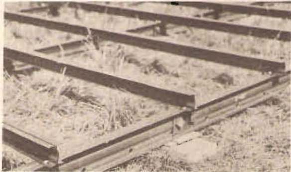
SILL AND JOISTS
