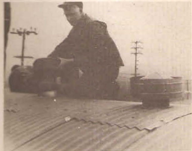
INSTALL SMOKE STACK
