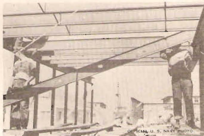
ERECT JOISTS
