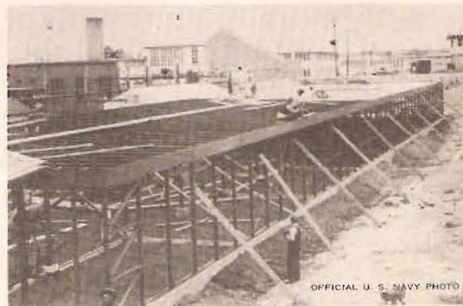
COMPLETE FLOOR FRAMING
