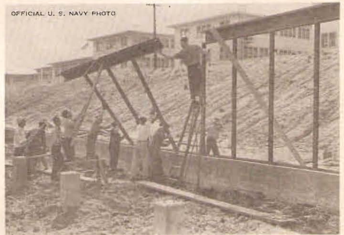
ERECT WALL SECTION
