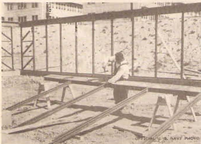
ASSEMBLE WALL SECTION
