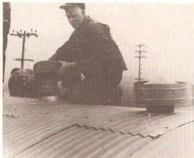
INSTALL SMOKE STACK
