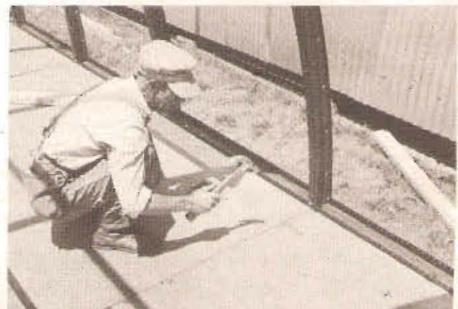
NAIL PANELS IN PLACE
