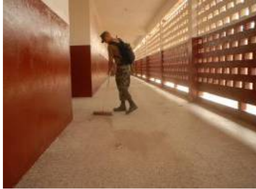
Cleaning up after work complete
