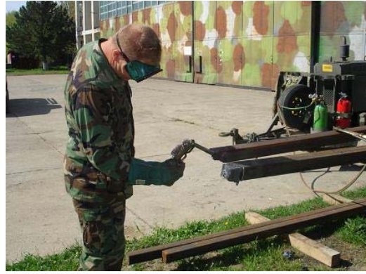
Seabee preparing steel for placement
