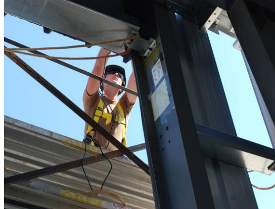
Crew member installing side paneling
