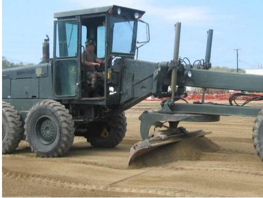
Grading and leveling the foundation of the K-Spans
