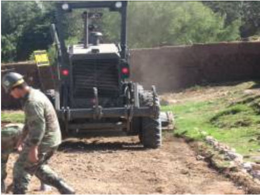
First grading pass of Volley ball/Soccer field
