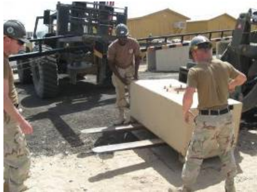
Seabees placing base of new arm-gate
