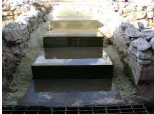
Finished steps from barracks to staging area
