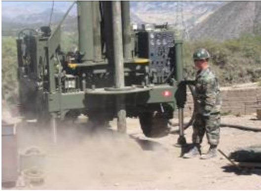
Breaking ground in Azangaro
