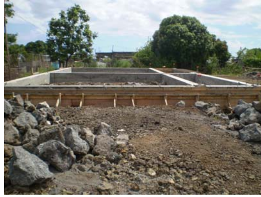
Complete rubble footer
