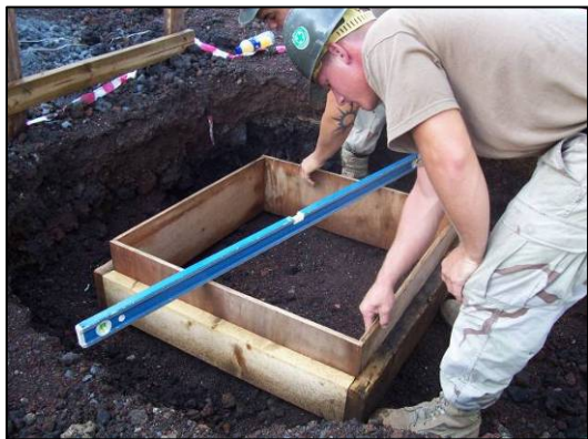
Figure 24 – Seabee setting forms for footers
