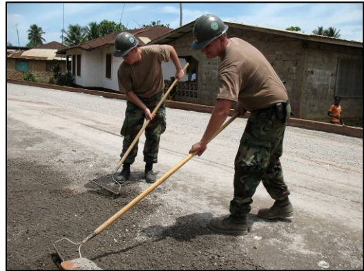
Figure 33 – Seabees working on side of road
