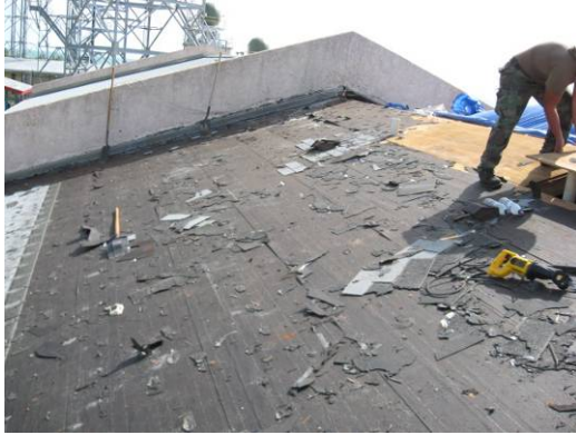
Seabee working on Roof Replacement
