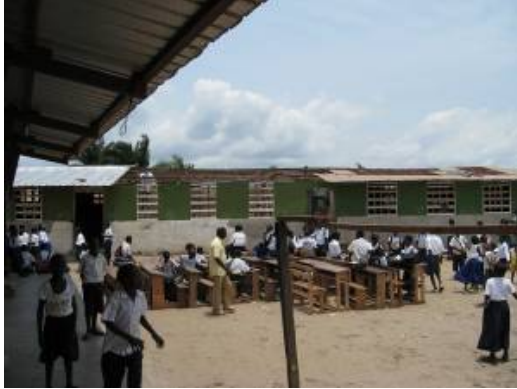
Repair of roofing section
