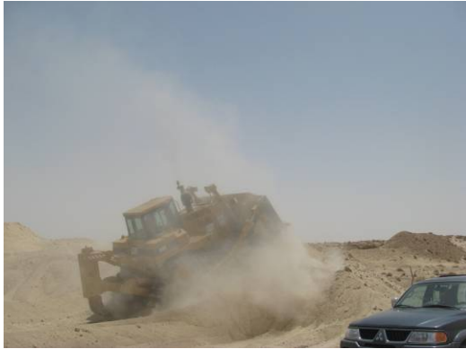
D-9 Dozer Constructing Berms
