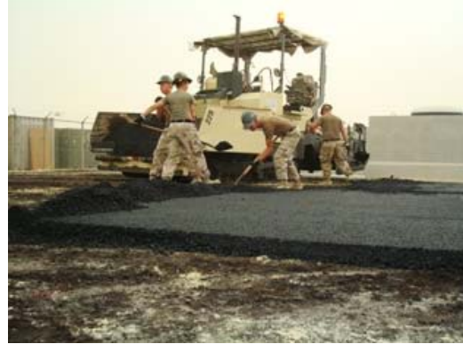
Seabees placing asphalt
