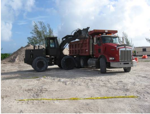
Removing existing concrete
