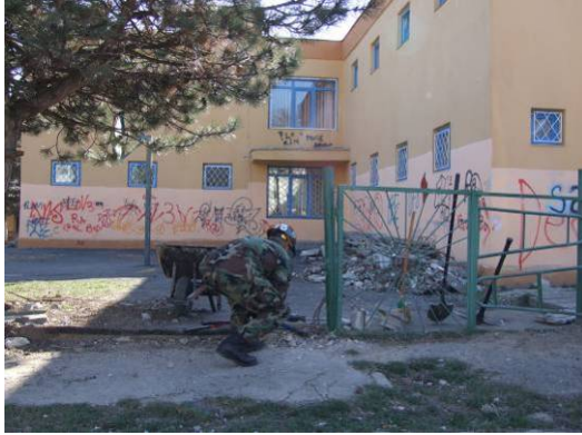
Removal of existing wall and gate
