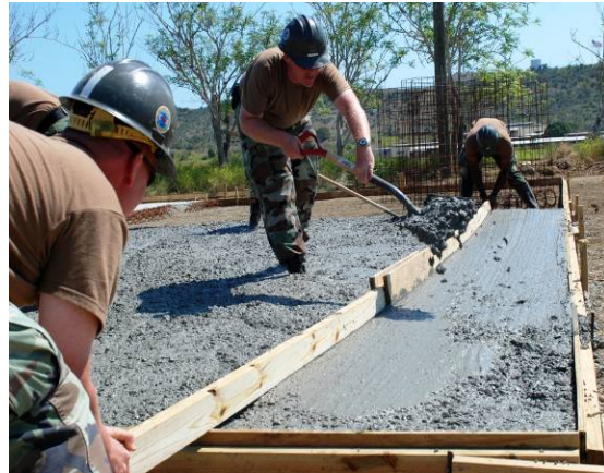
Crew working second portion of pad for NAVSTA GTMO MWR
