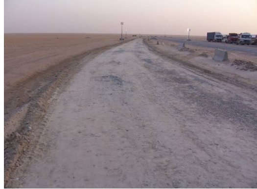
Completed TAA road section
