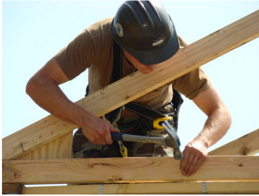
Connex Box Roof Construction
