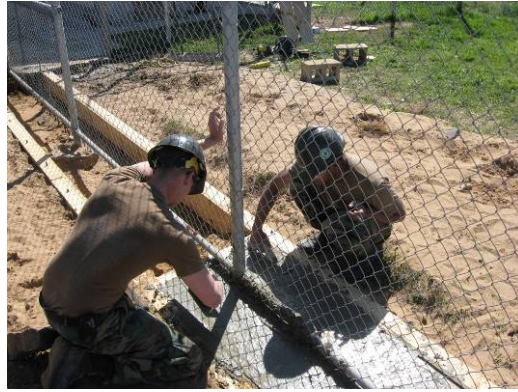
Seabees placing concrete footer
