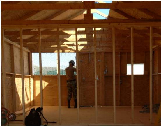
Interior of SWA Hut constructed for Joint Task Force Guantanamo
