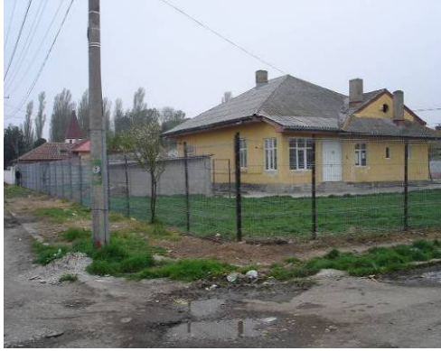
Outside overview of completed fencing
