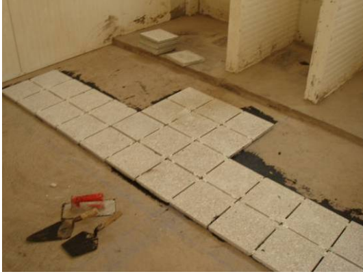
Latrine tile installation
