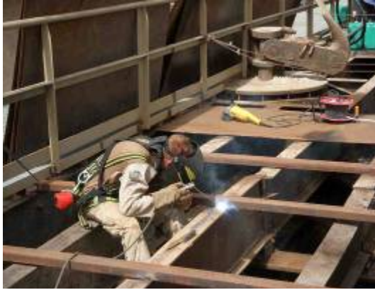
Welding beams for trash containment area
