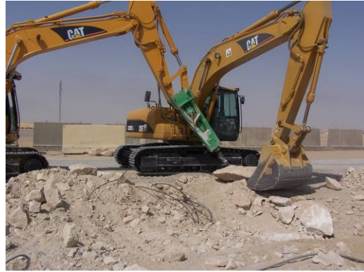
Removing boulders from proposed trench
