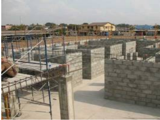
Installing rebar at turnover
