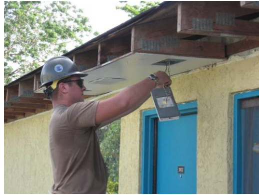
Disconnecting exterior lights
