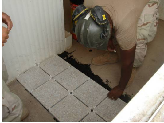
Dormitory tile installation
