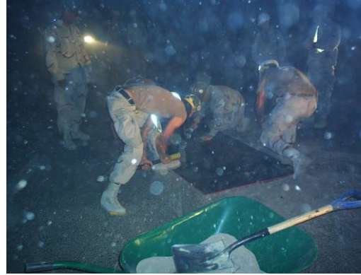
Placing plywood on top of pothole
