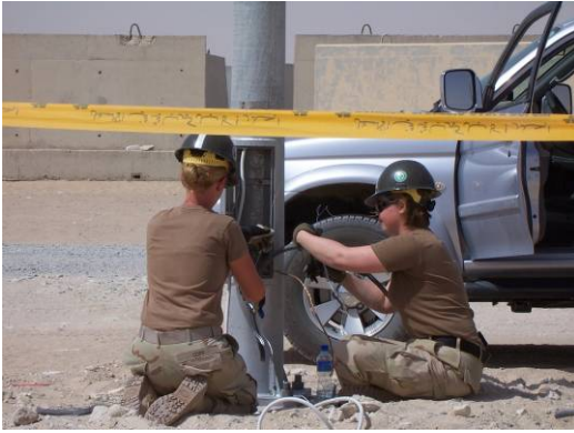
CE's making final connection to pole
