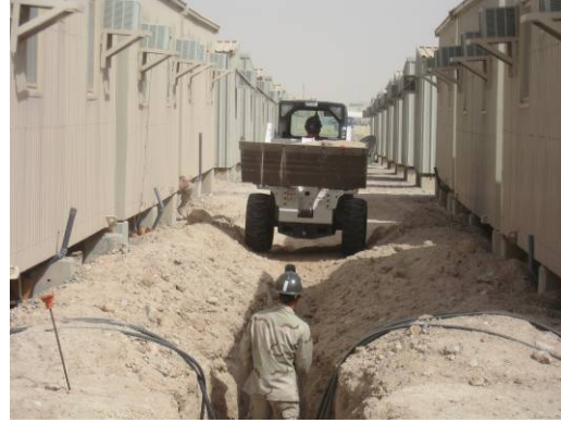
Backfilling sewer line
