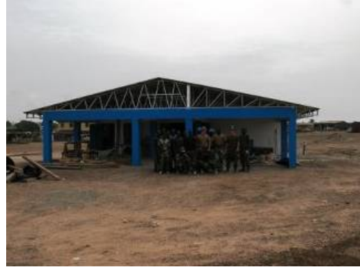
Clinic exterior at completion
