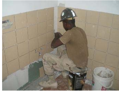
Placing ceramic wall tile
