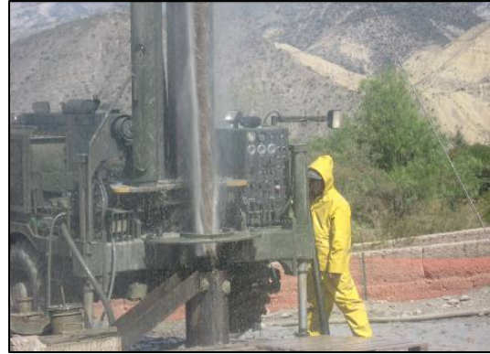
Figure 41 – Blowing the hole for Water Well Peru
