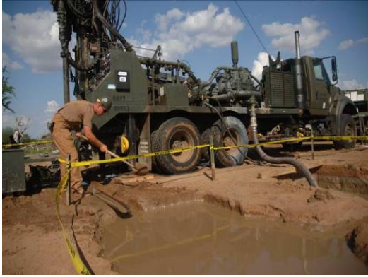
Well drilling operations
