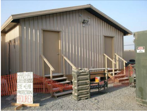
Completed SWA Hut
