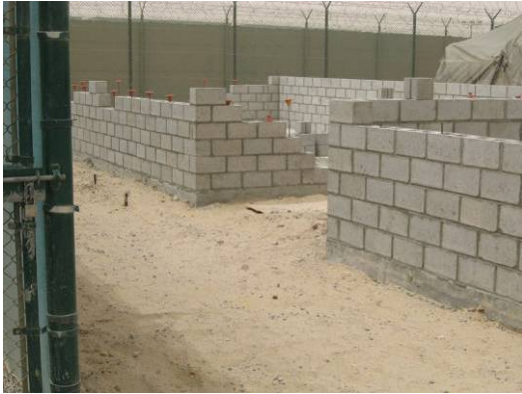
Echo Pad CMU Walls In Progress
