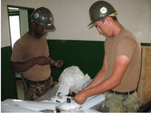
Installing ceiling fans
