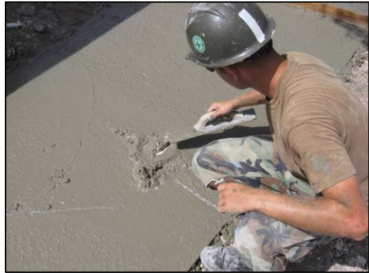
Figure 35 – Seabee placing concrete for sidewalk
