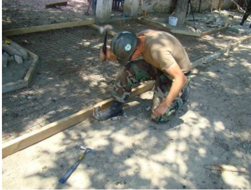
Seabee forming for new sidewalk
