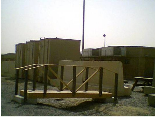
Bridge set over drainage ditch
