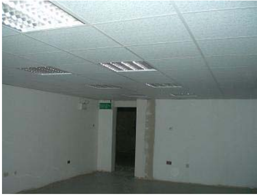
Finished drop ceiling
