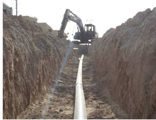
Placing 4" main water line
