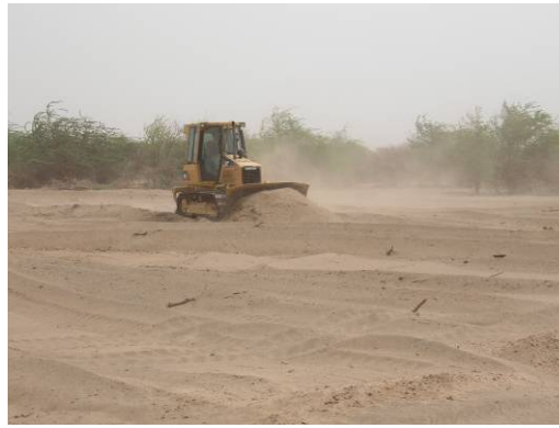
Earthwork in camp expansion area
