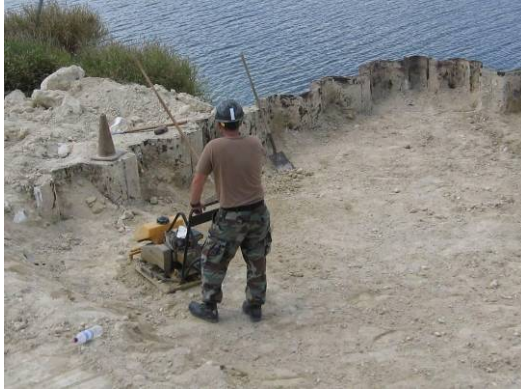
Soil Compaction on the bridge abutment
