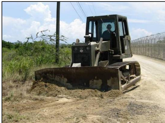
Figure 37 – Working on perimeter road
