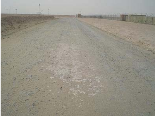
Grading perimeter road
