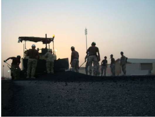
Seabees starting the 2 nd lift on Phase V
