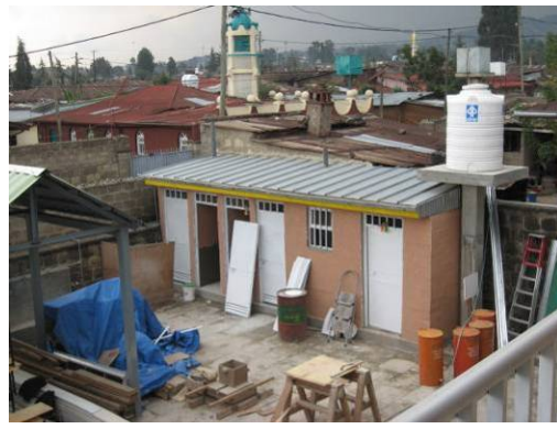
Latrine and new cistern
