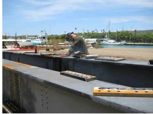
Completing a top weld on the Windward beams
