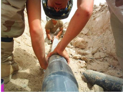
Gluing 4" sewer line together
