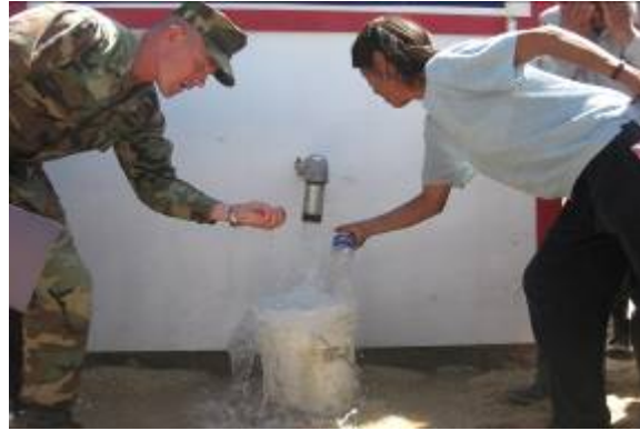
Water discharging at 17 GPM from completed well
