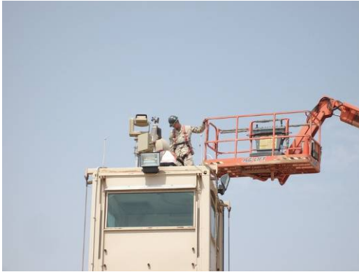
Installing photo cells
