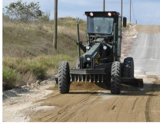
Grading operations along Perimeter Road
