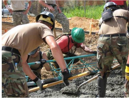
Seabees placing concrete
