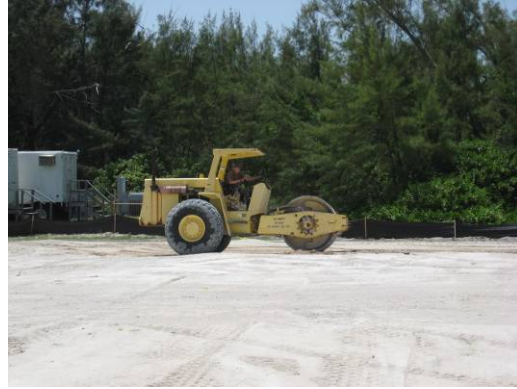
Compacting fill material
