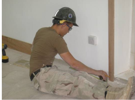
Crew member installing trim
