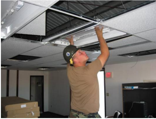
Installing drop ceiling
