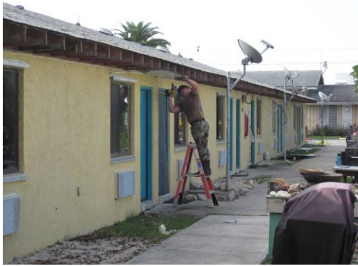
Removal of soffit and fascia
