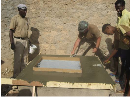
Water distribution point repair
