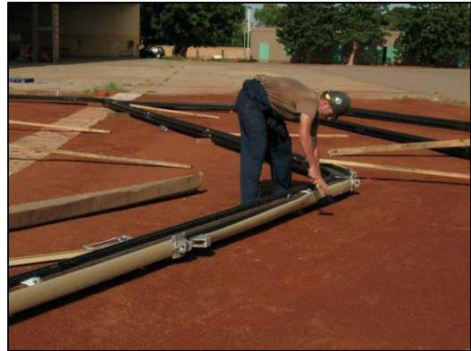
Figure 32 – Seabees assembling arches for LAMS
