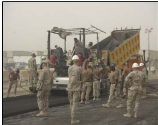
Figure 48 – Contractor delivering asphalt
