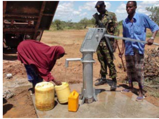
Completed Shaba well
