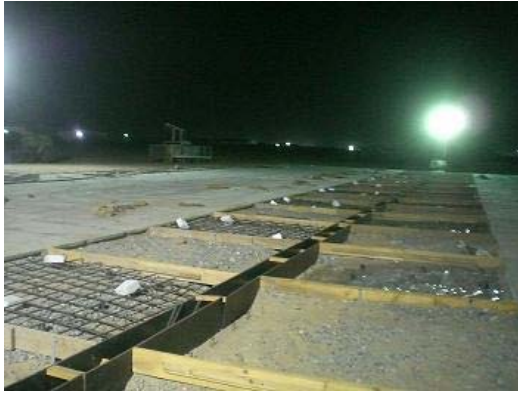
Forms in place
