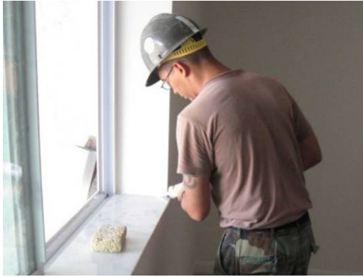
Installing window sills
