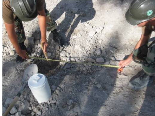
Layout for sidewalk
