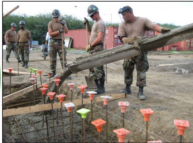
Figure 13 – Seabees placing concrete
