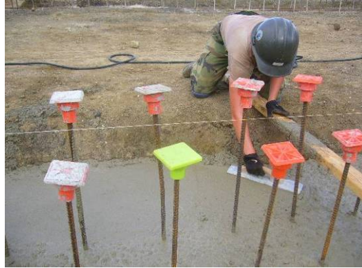
Seabee finishing concrete for foundation
