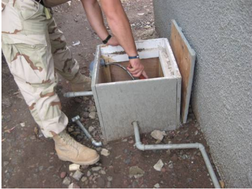
Repairing water pump
