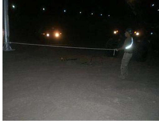
Guide rope for setting poles
