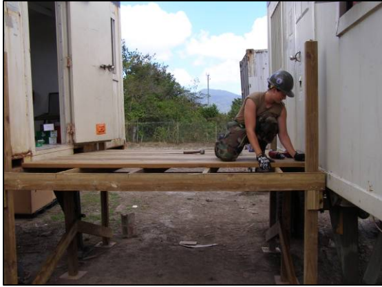
Figure 40 – Building a Platform
