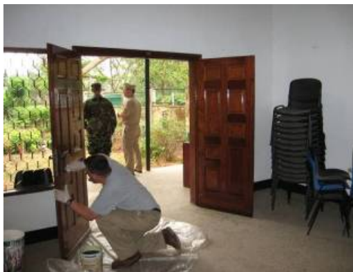
Painting and staining walls and doors
