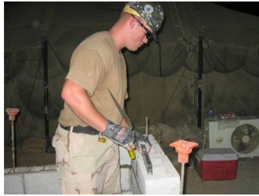
Placing CMU Block
