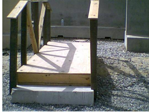
Bridge set over drainage ditch
