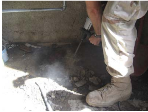
Demolishing concrete slab
