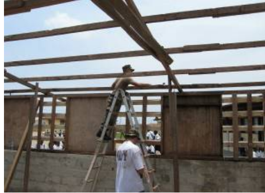
Fort McHenry Sailor holding ladder during repair
