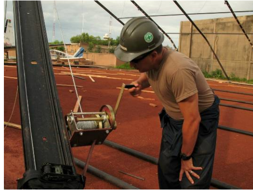
Winching arches up
