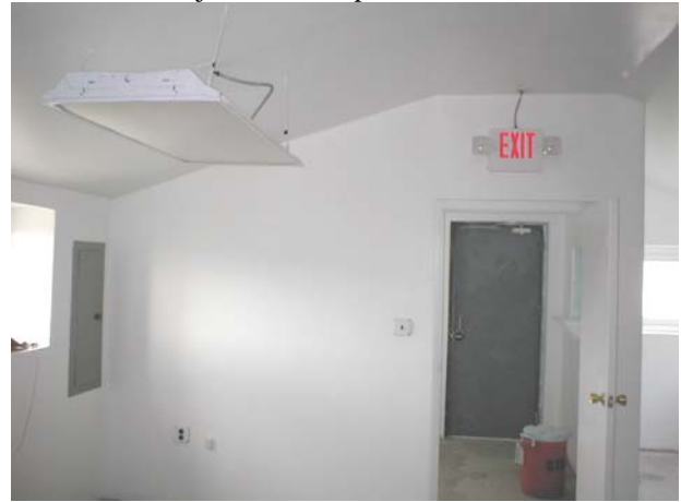
LEFT: Project at turnover. BOTTOM: Project near completion.
