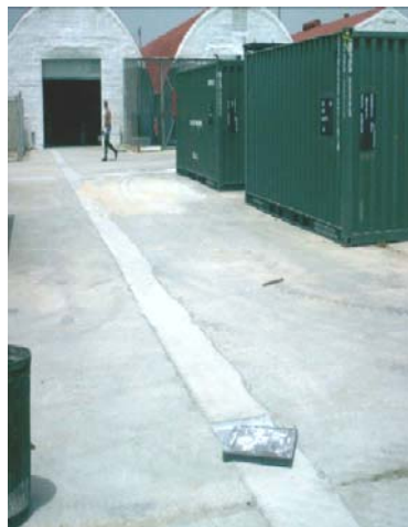
Completed LAN cable run
