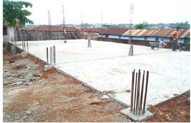
LEFT: Pre-construction site condition BOTTOM: Tasked 50% completion of Nima Community Center
