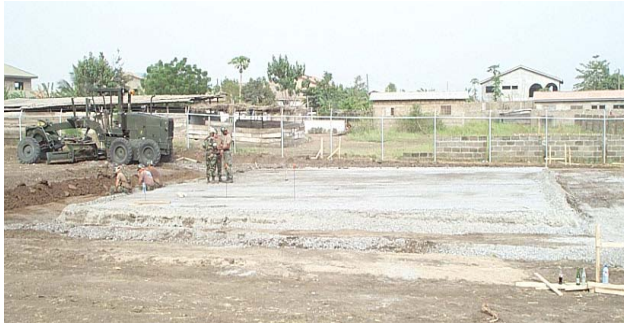
LEFT: Footprint of building graded to elevation BOTTOM: Completed Haatso Medical Clinic
