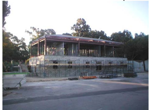
BOTTOM: First floor block and stairwell complete.
