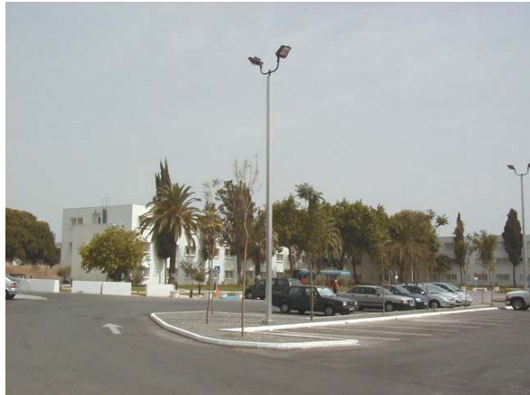
Repair Light Pole at BOQ 39
