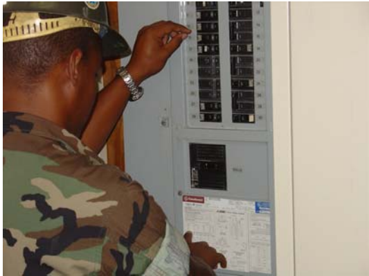
CE3 checks an electrical panel in MLO.
