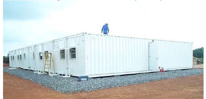
BOTTOM: Completed 64-man dormitory facility
