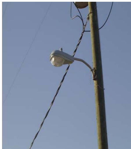
Replace and upgrade camp exterior
