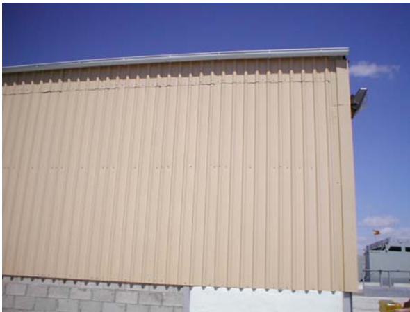
Finish Sheet metal at Fuel Skimmer Shed
