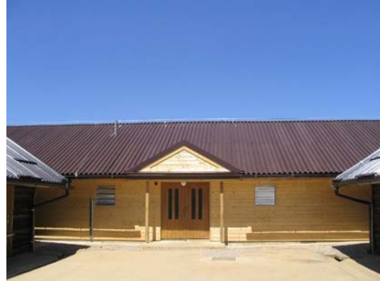
LEFT: Latrine site at turnover BOTTOM: Front of Latrine at completion
