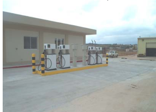
LEFT: MORGAS station at turnover. BOTTOM: MORGAS station at completion.
