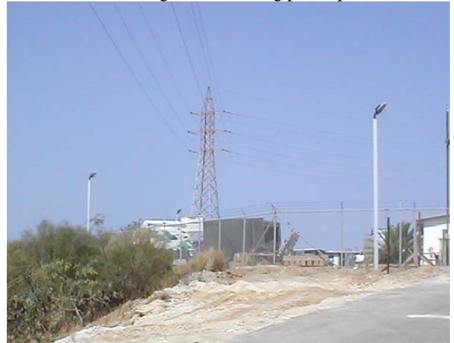
LEFT: Light # 5 during operational test. BELOW: View of lights surrounding power plant.
