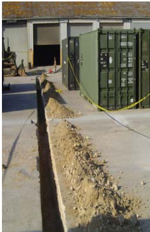
Open trench for LAN cable
