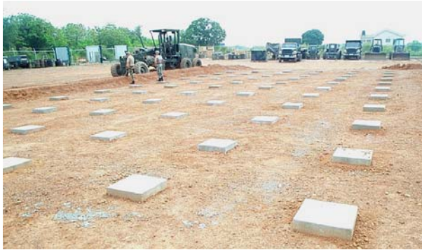
LEFT: 66 individual foundation piers for modular units
