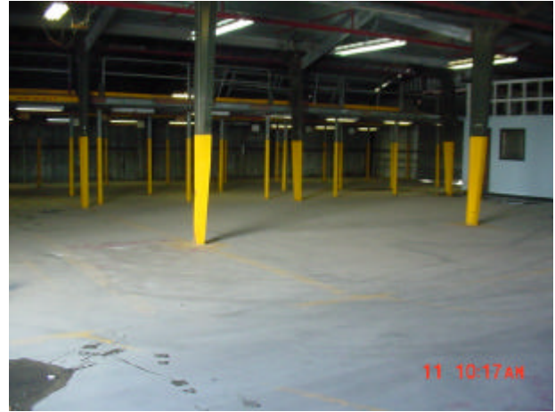
MLO Warehouse ready for turnover
