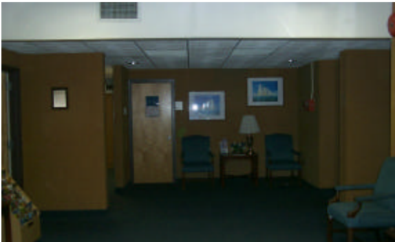
Replaced ceiling tile in all common areas BEQ U-112
