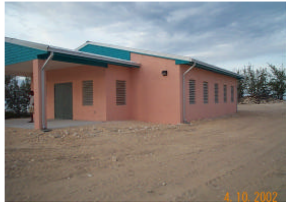
Completed Exercise Control Facility
