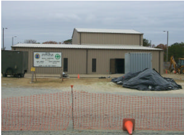
Exterior of building completely enclosed with all doors and windows installed
