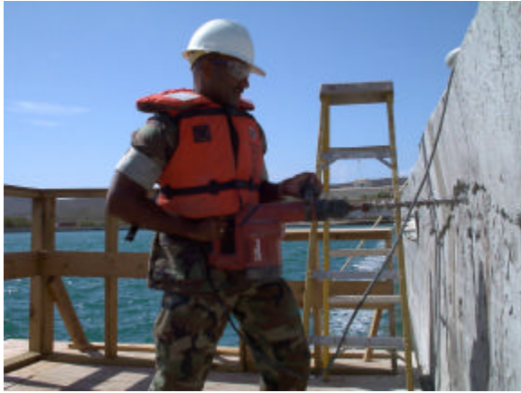
Working on side of Pier Alpha
