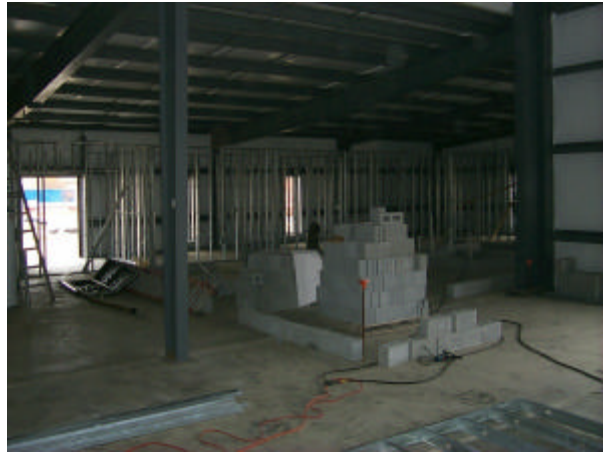
Installation of metal stud walls to be finished with drywall
