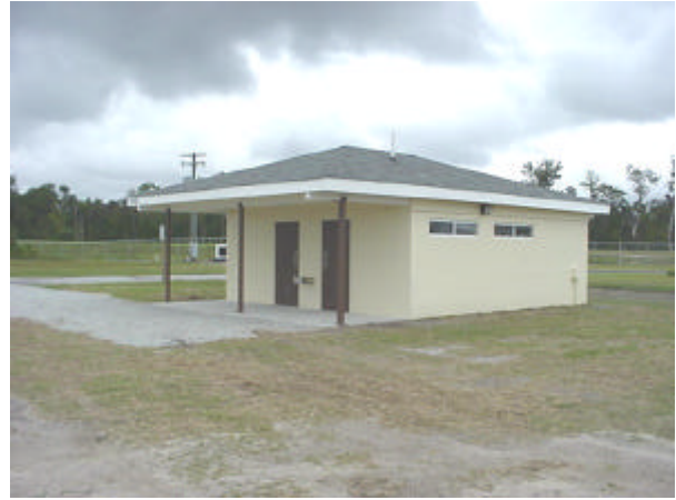
Finished SOI Head Facility
