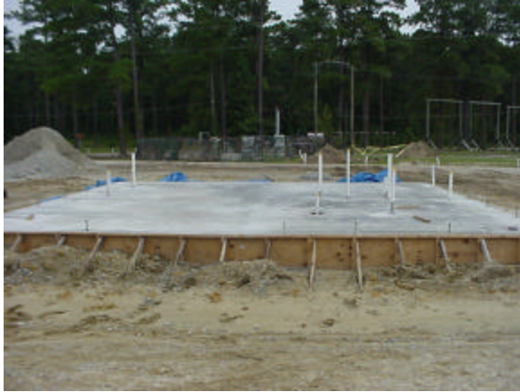
Newly placed thickened slab
