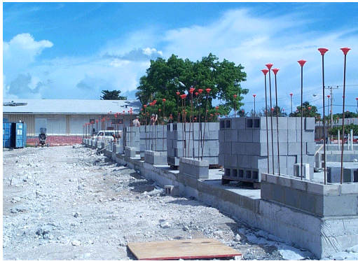
CBH-11 in progress
