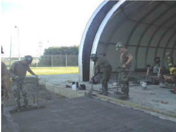
Placing concrete for TFS Ramp
