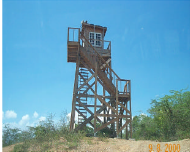
Observation tower after construction of new stairs
