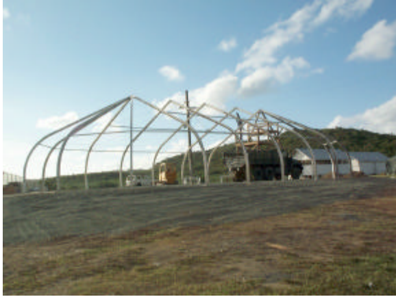
TFS construction in-progress
