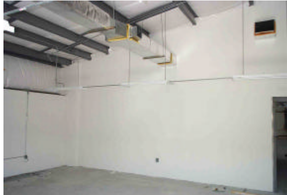
Finished interior and installed duct work
