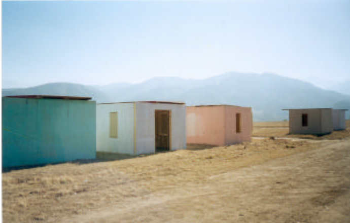
Simulated Villages Construction in progress
