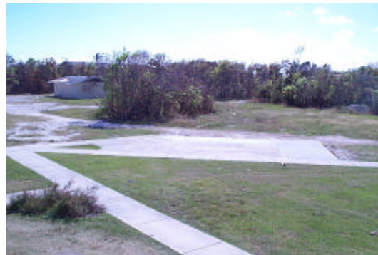
Construct new concrete pad
