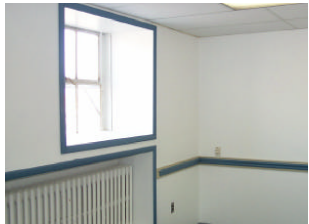
Renovation of office spaces for Air Group at LP-4
