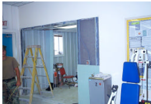
Wall removal in base gym
