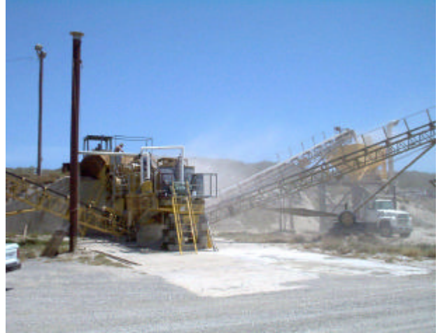
Crusher – Quarry Center
