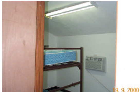
Renovated BEQ room
