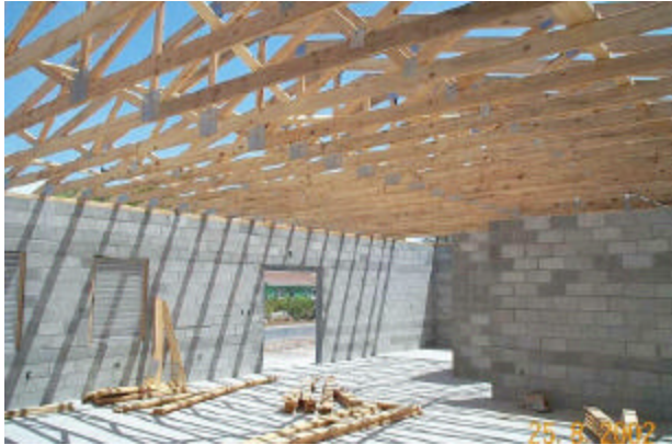
Community Center under construction
