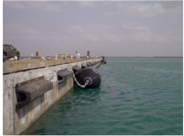
Pier Alpha Fenders installed
