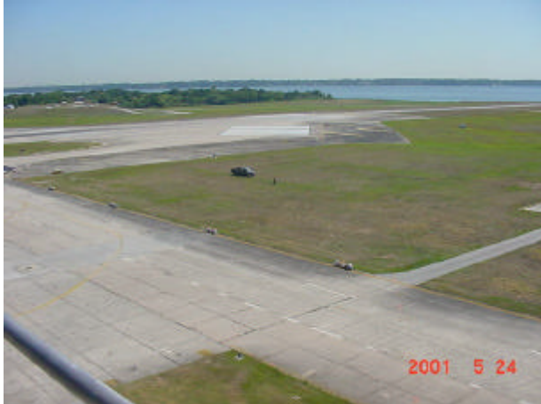
North end of Taxiway Bravo Expansion.
