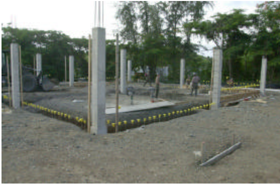
Above and Right: Construction in progress
