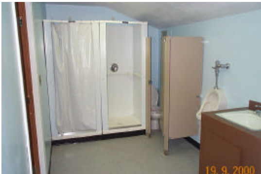
Renovated BEQ bathroom
