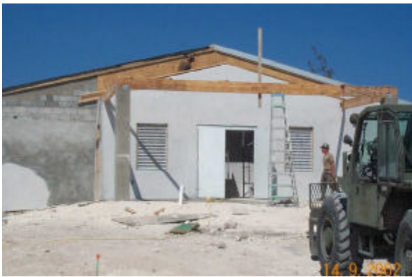
Exercise Control Facility in construction
