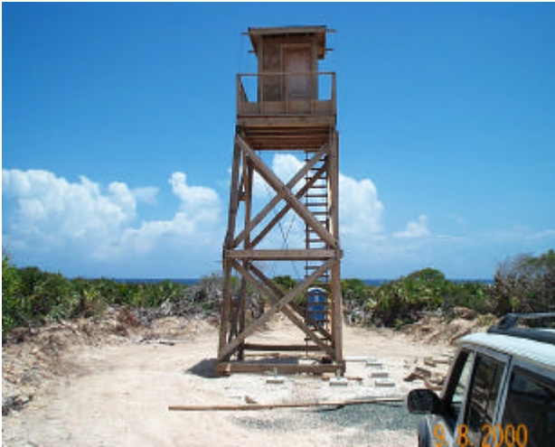
Observation tower before construction of stairs
