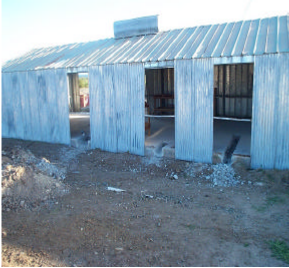
Galley prior to renovation
