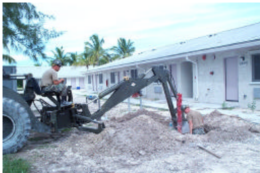
Water line repairs
