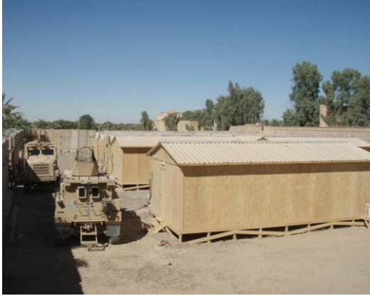
Completed SWA Huts
