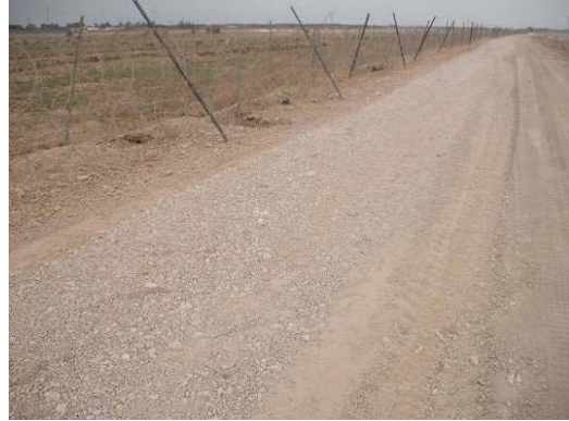
Repaired section of road
