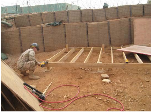
Decking construction
