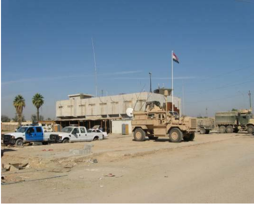
JCC District HQ Facility
