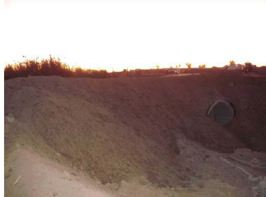
New culvert and road elevation
