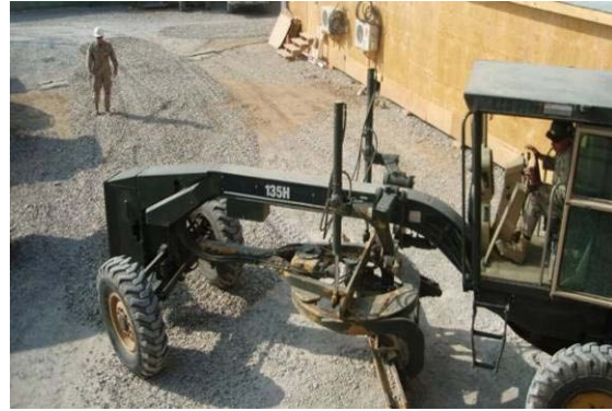
Camp Gravel Spreading
