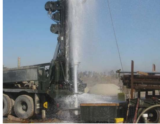
Air developing the Well
