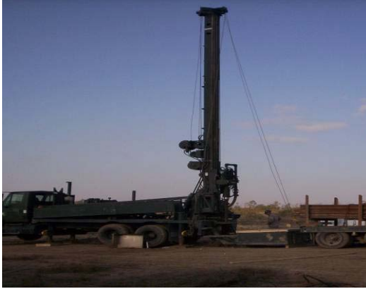
Drilling for water
