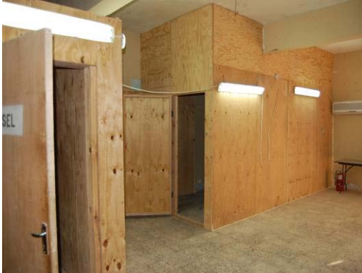
Partition section complete
