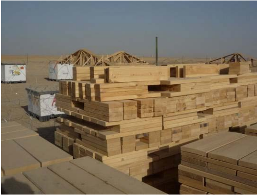
550 Pre-fabricated footers palletized
