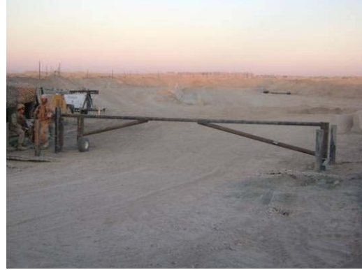
Installed swing arm gate
