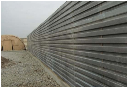
Concrete Pad Placement
