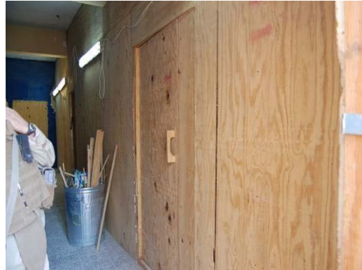
Wall partition with access door
