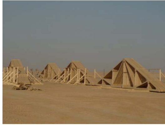
121 Pre-fabricated Trusses stacked and braced
