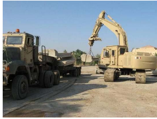
Loading T Walls for Placement
