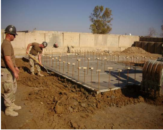
Finished Concrete Pad
