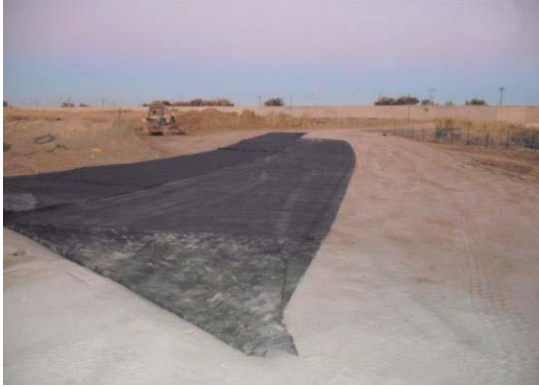
Geotextile fabric placement
