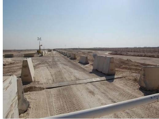
Jersey Barrier placement
