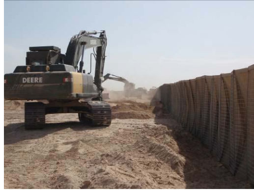
Placing Hescos for the temporary ECP
