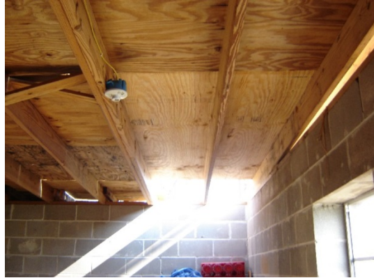
The interior of the facility as electrical repairs are in progress.
