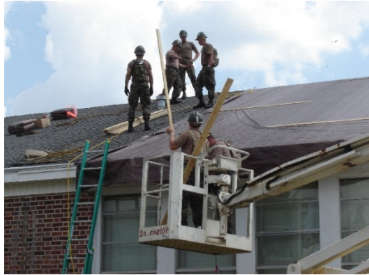
Crew applying tarps to the roof at Rocky Creek Elementary School
