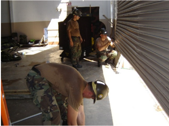
A crew from NMCB-7 works to repair a large roll-up door.
