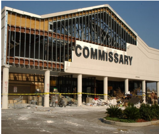
Front view of CBC Gulfport commissary
