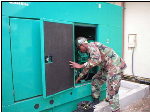
Installing a new backup generator
