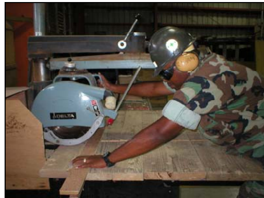
Making a finish cut on door trim
