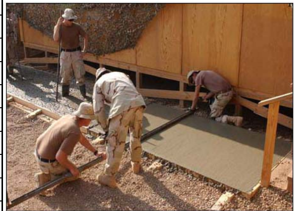
PLACEMENT OF CAMP SIDEWALK
