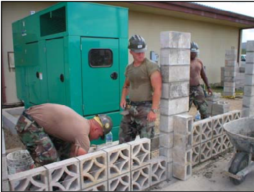
Laying blocks on the generator pad project.
