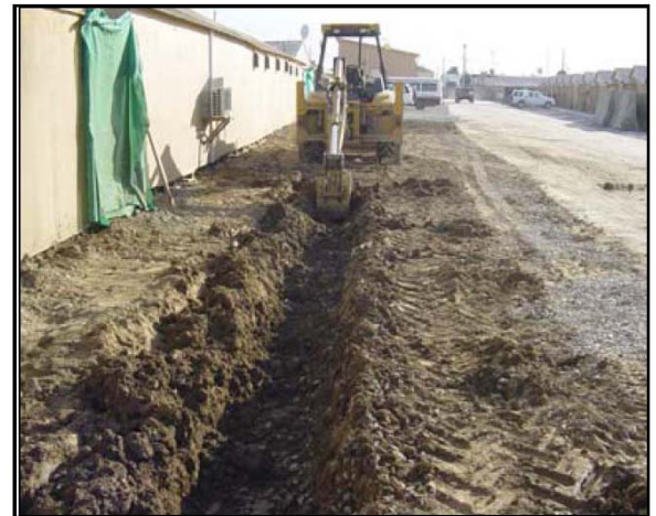
COMPOUND FENCE TRENCHING
